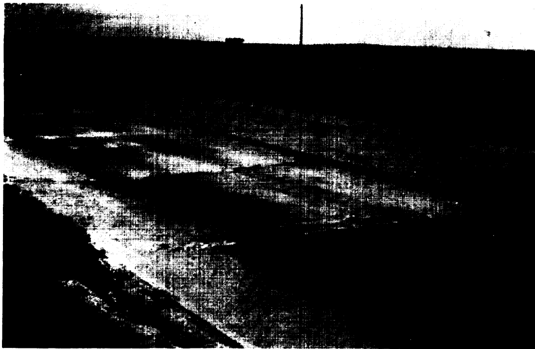
Figure 78 Example of Pavement Distress Caused by Water Under Pavement
