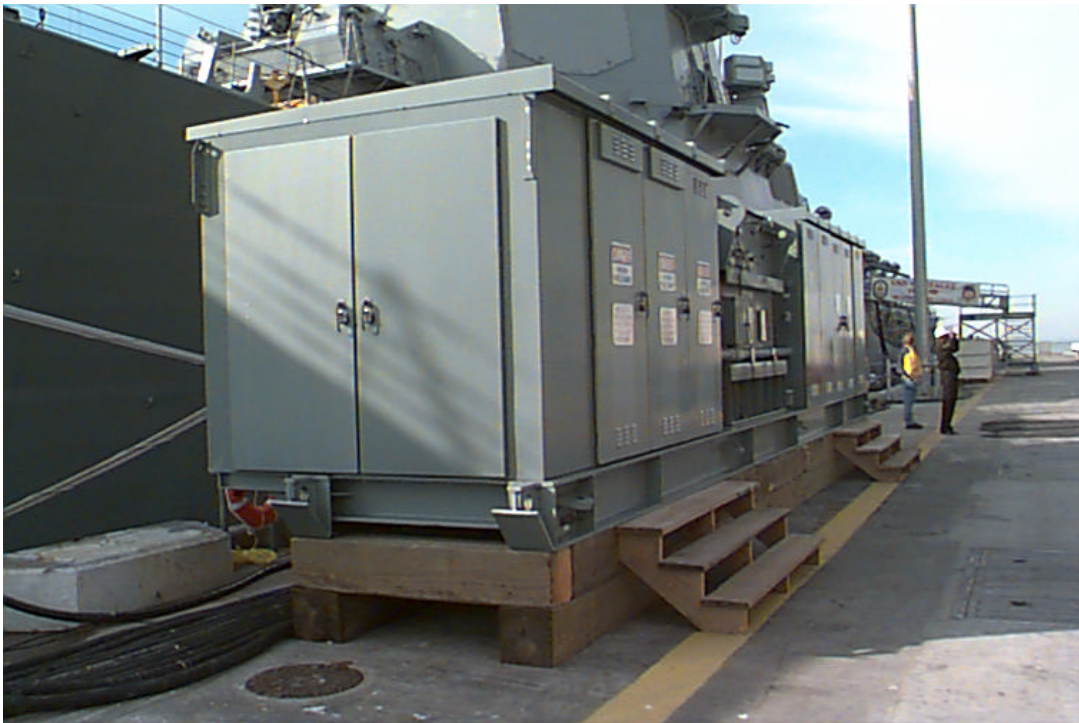
Picture C. A skid-mounted substation
