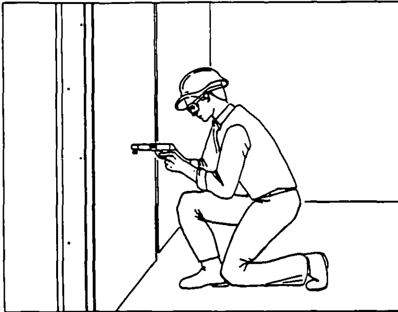
Figure 10. Installation of laminates using powder-driven fastener.
