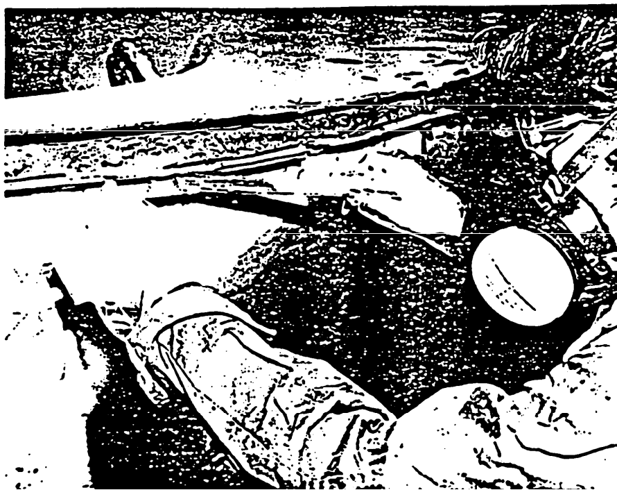
FIGURE 21. Applying resin paste to edge delamination.
