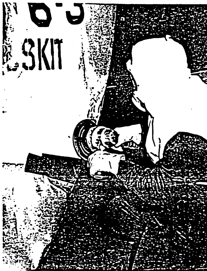
FIGURE 49. Removing high spots with power sander.
