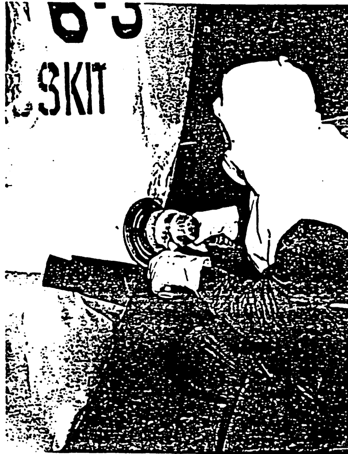
FIGURE 49. Removing high spots with power sander.
