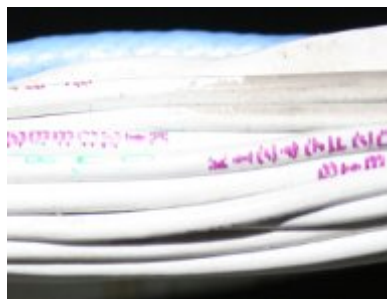
Acceptable Insulation is not damaged, chafed or flaking.
