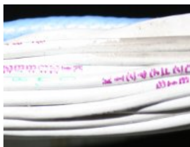
Acceptable Insulation is not damaged
