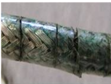
Unacceptable Radial crack in the insulation.
