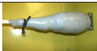
Acceptable Dual wrap kit installed properly using self- leveling green, stretch seal (inner, pink layer) and self-fusing silicone tape (outer, gray layer), secured with lacing tape.
