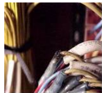
Unacceptable Overheating seen at the splice termination.
