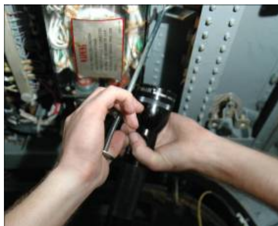
Acceptable Proper use of a mirror and flashlight inspecting a wiring harness.
