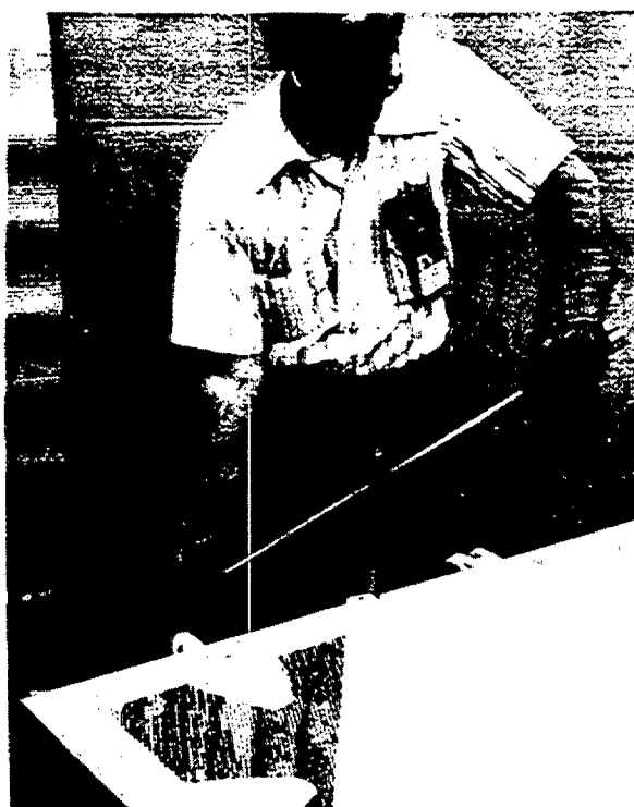
b. Peeling Sandwich Skin With "Can Opener" Type Tool
