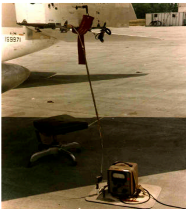
FIGURE 20. Voltage-Ground Measurements Setup
