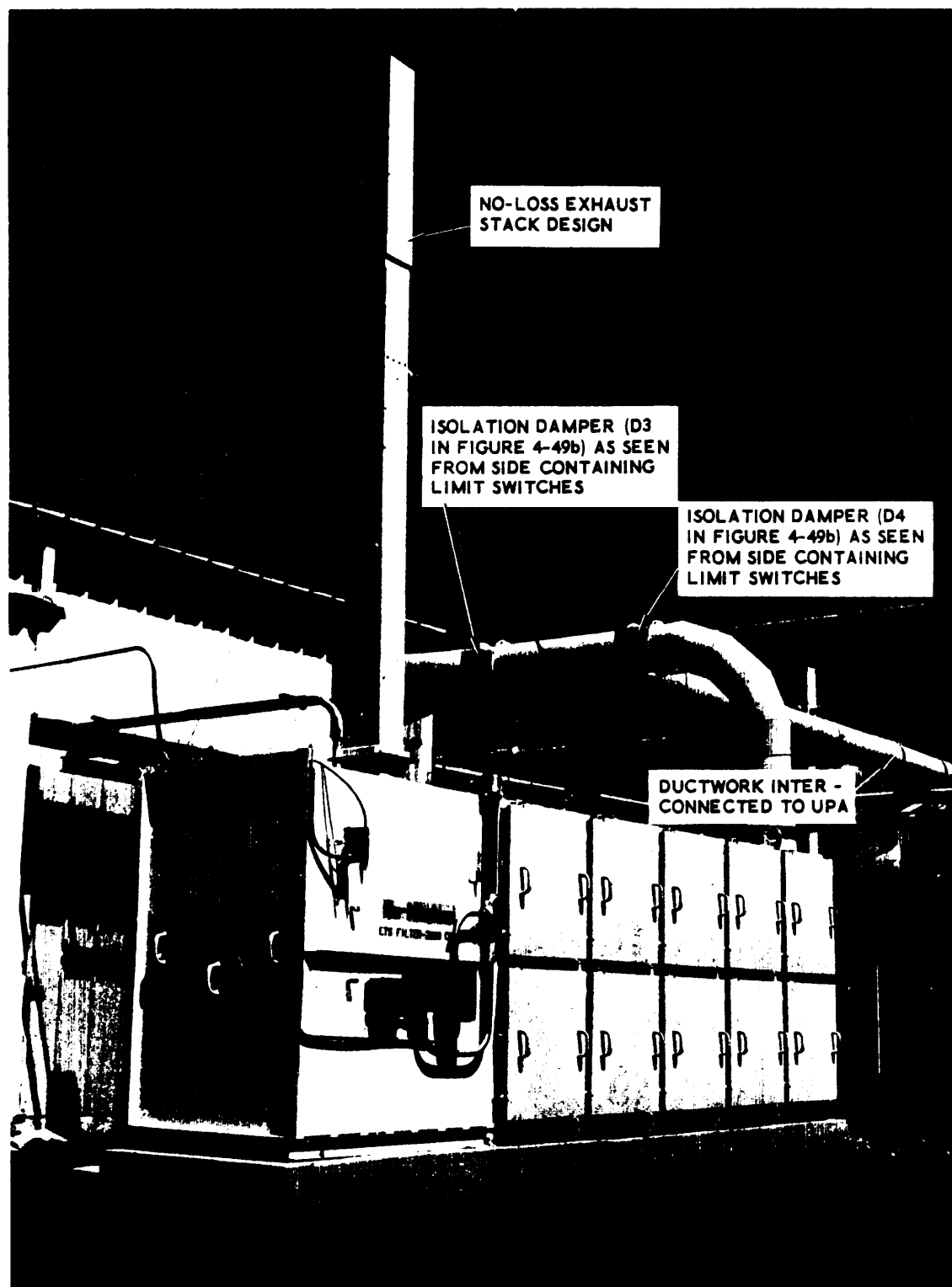
Figure 4-51. Type I Filter System (2,000 Cfm) For Explosive Treatment System At CAMDS Showing Isolation Dampers And Interconnecting Ductwork
