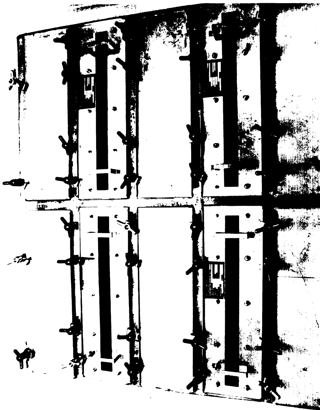
Figure 4-21. Bank Of Adsorber Trays And Blankoff Plates Using Captive-Nut Clamps. This Is 3,000 Cfm Arrangement In 6,000 Cfm Type II Filter System
