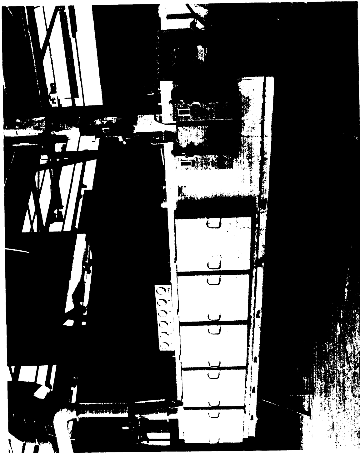
Figure 8-7. Front View Of 666 Cfm Glovebox Ventilation System For DATS
