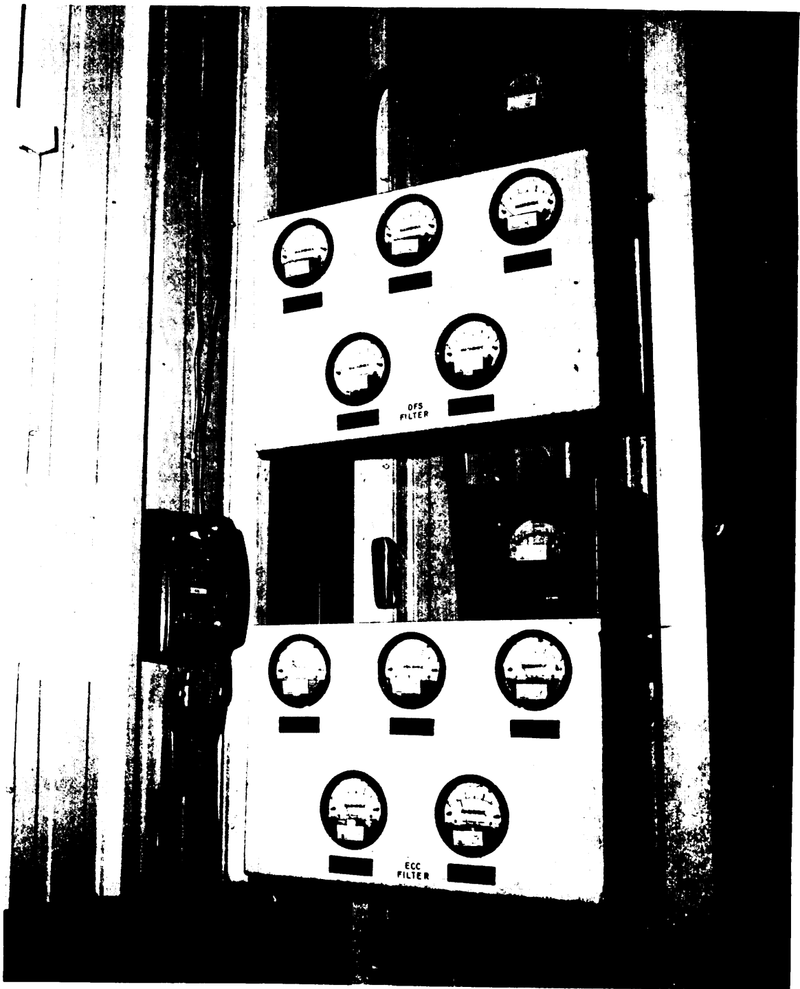
Figure 4-28. Remote Indoor Instrument Station For CAMDS Filter System
