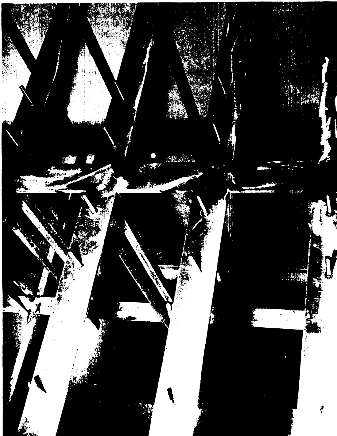
Figure 4-17. Mounting Frames In Type II Filter System (6,000 Cfm). Adsorber (Bank No. 4) Mounting Frames Are In Foreground And HEPA Filter Mounting Frames (Bank No. 5) Are In Rear
