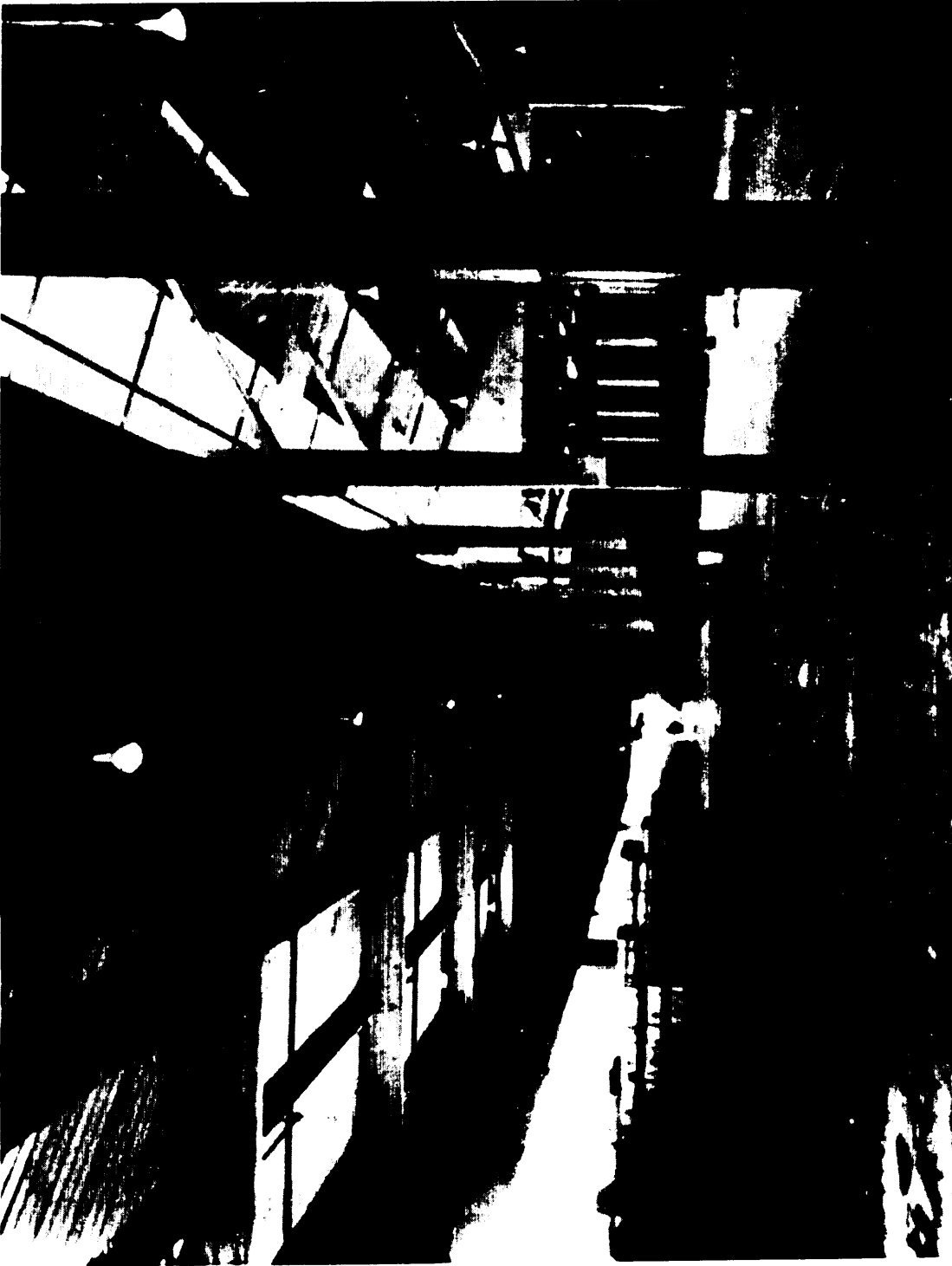
FIGURE 38. Glued laminated timber beams and columns utilized in a warehouse.
