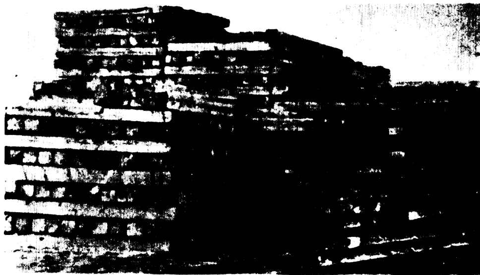
B. Railroad ties solid piled by 11-by-11 method-11 ties in each layer.
