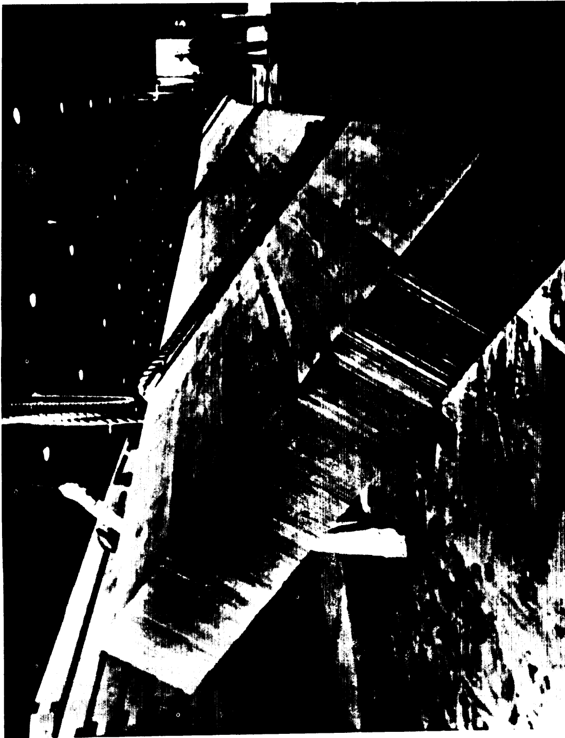
FIGURE 37. Glued-laminated timber beam, 97 feet long.
