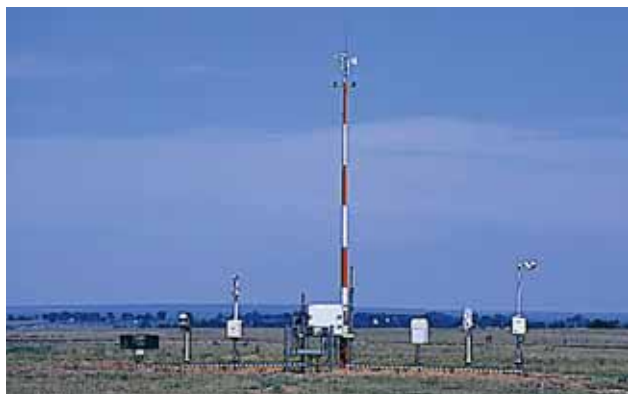
Figure 2-12. ASOS Station Installation.
