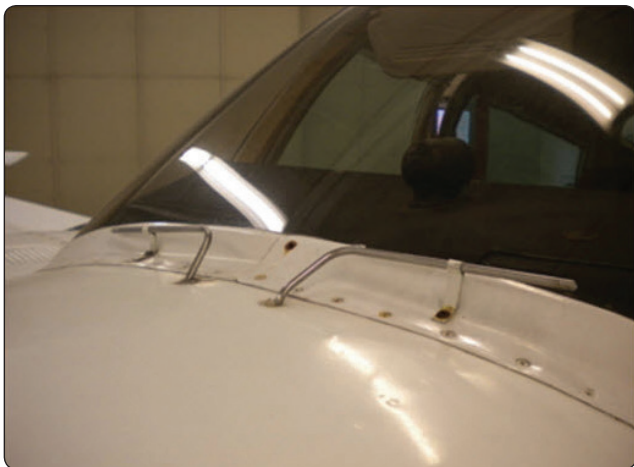
Figure 15-46. Chemical deicing spray tubes.
