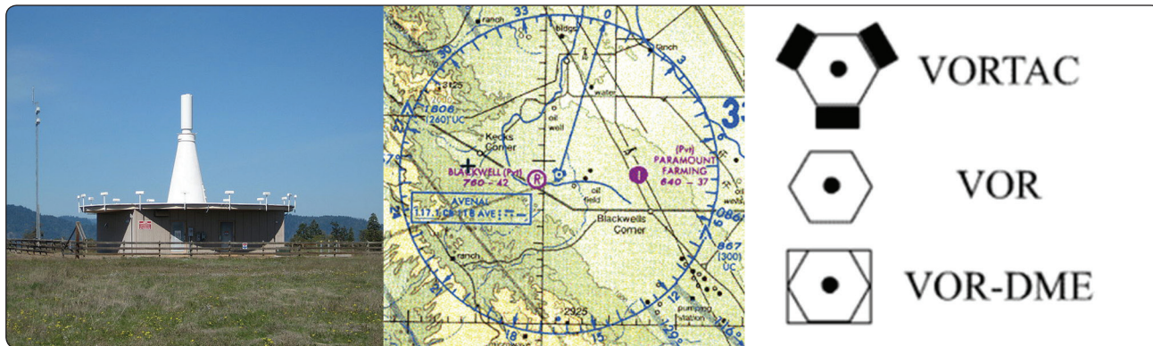
Figure 11-95. A VOR ground station.
