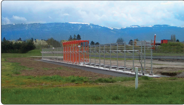
Figure 11-111. An ILS localizer antenna.
