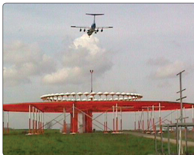
Figure 11-119. A VOR with DME ground station.
