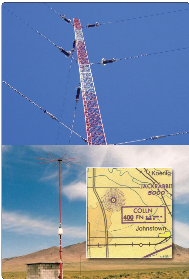
Figure 11-106. Nondirectional broadcast antenna in the LF and medium frequency range are used for ADF navigation.
