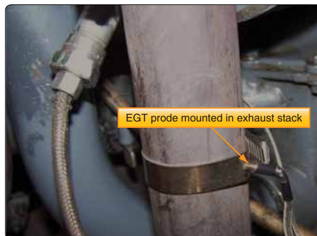
Figure 6-60. EGT probe in exhaust stack.
