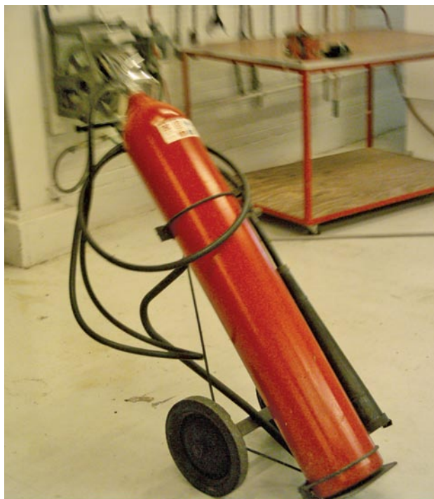
Figure 11-4. Carbon dioxide fire extinguisher.
