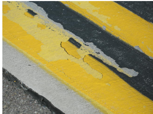
FIGURE 2-1. PEELING PAINT LAYERS
