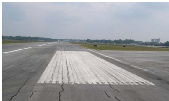
FIGURE 4-17. AFTER WATERBLASTING, BUT BEFORE PAINTING.
