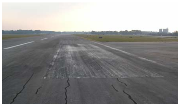
FIGURE 4-16. BEFORE WATERBLASTING: ALGAE OBSCURE MARKING.
