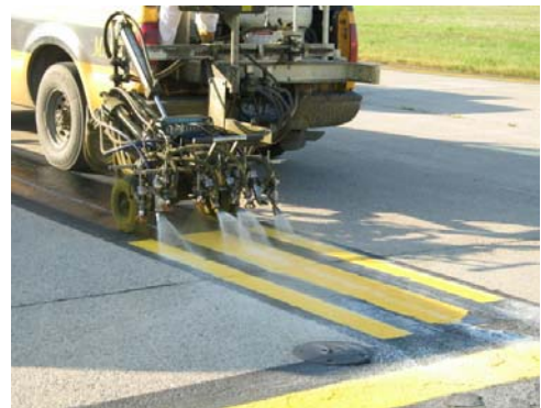
FIGURE 6-23. THREE PAINT GUNS AND FOUR BEAD GUNS APPLIED THE YELLOW PATTERN IN ONE PASS.
