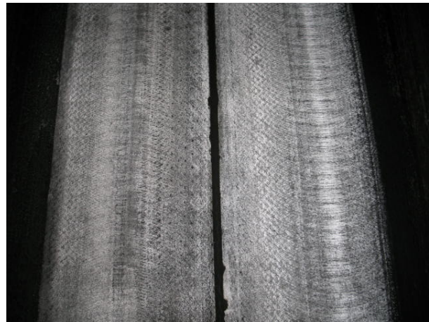
FIGURE 4-40. HEAVY RUBBER DEPOSITS WERE REMOVED FROM THIS CENTERLINE MARKING WITH ULTRA HIGH-PRESSURE WATERBLASTING.
