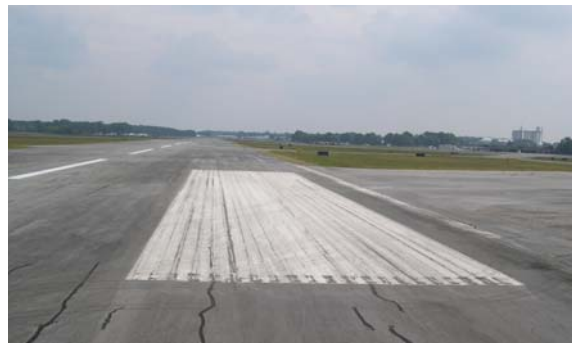
FIGURE 4-17. AFTER WATERBLASTING, BUT BEFORE PAINTING.
