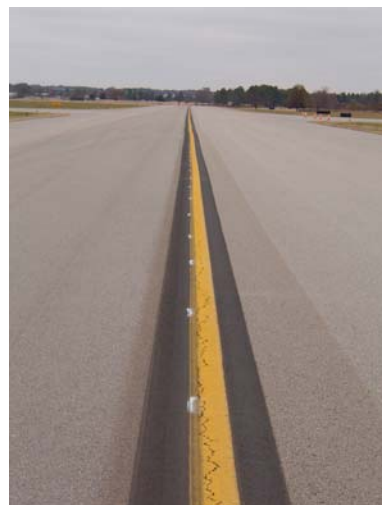
FIGURE 6-4. LAYOUT WITH PAINT SPOTS TO STRAIGHTEN EXISTING MARKINGS.
