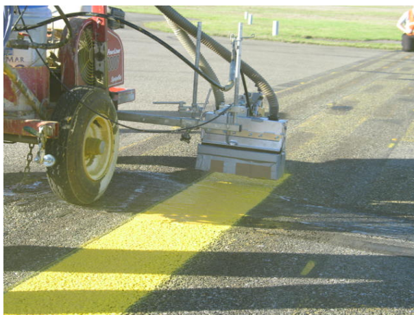
FIGURE 6-40. GLASS BEAD DISPENSER HAS BEEN MODIFIED WITH A CARDBOARD WINDSCREEN.
