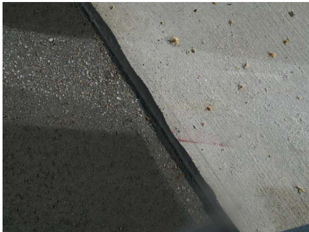
FIGURE 5-14. USED FOR REMOVAL ON NON-GROOVED SURFACES, SHOTBLASTING CAN BE A BEST PRACTICE.
