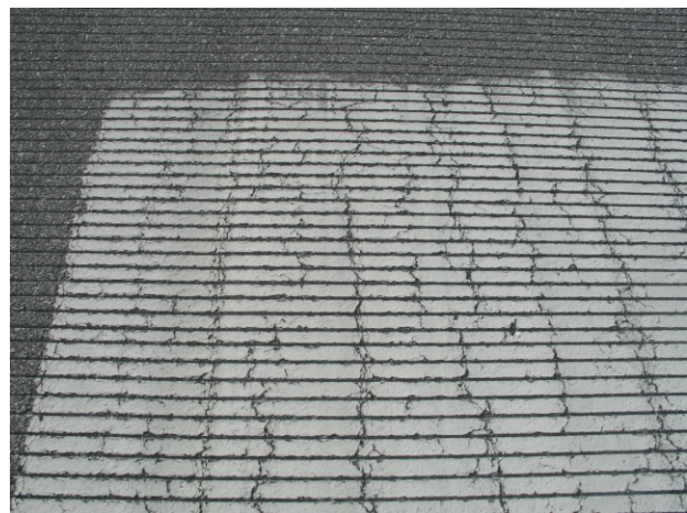
FIGURE 6-12. THE HEAVIER PAINT IN THE OVERLAP AREA CAUSED THE PAINT AND THE ASPHALT TO CRACK.
