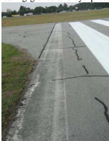
FIGURE 4-14. WATER FROM THE AIRPORT'S FIRE TRUCK, WITH 150 PSI, RINSED THE SIDELINE.
