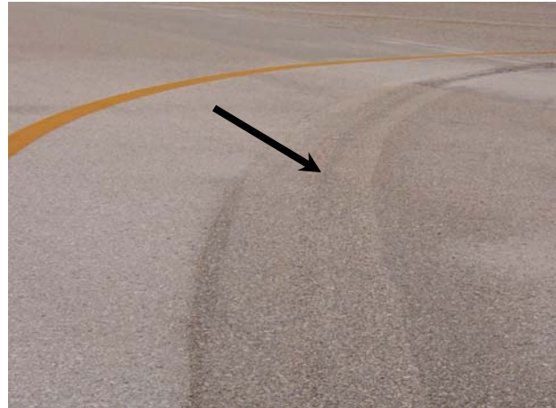
FIGURE 5-19. REMOVAL DONE ONE YEAR EARLIER; THE DARK SCAR HAS OXIDIZED AND FADED.
