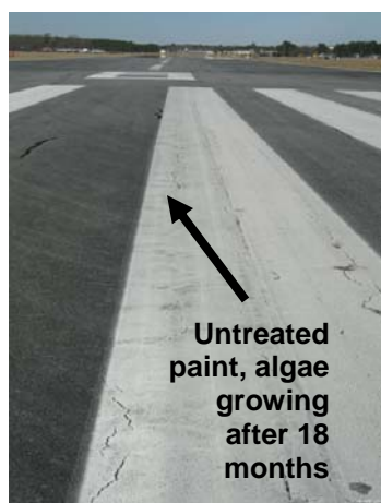
FIGURE 4-18. PAINT USED WAS STANDARD TT-P-1952E.
