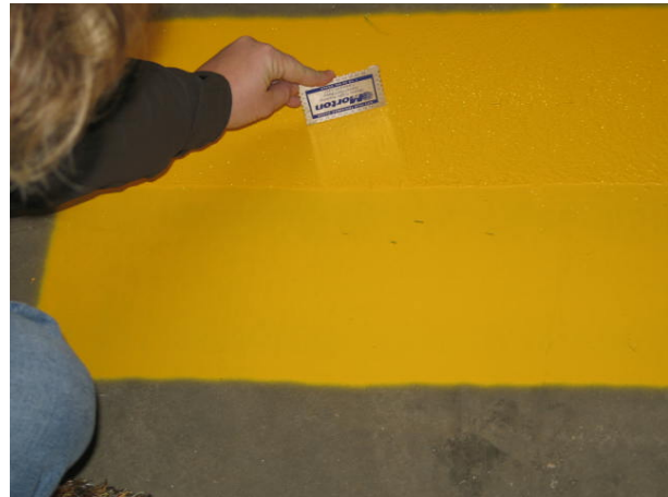
FIGURE 6-62. USE OF WET FILM GAUGE.
