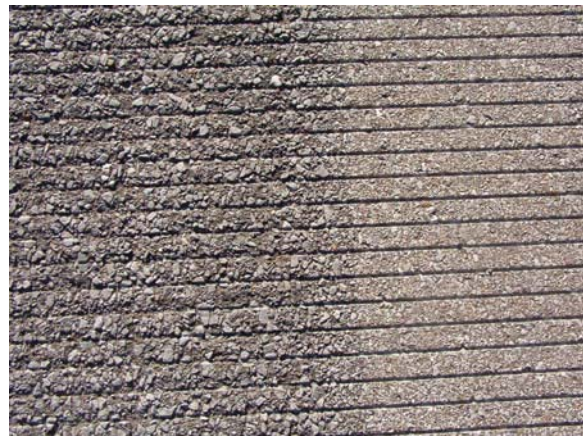
FIGURE 2-6. RESULTS OF WATERBLASTING REMOVAL ON POOR ASPHALT SEEN IN FIGURE 2-5.
