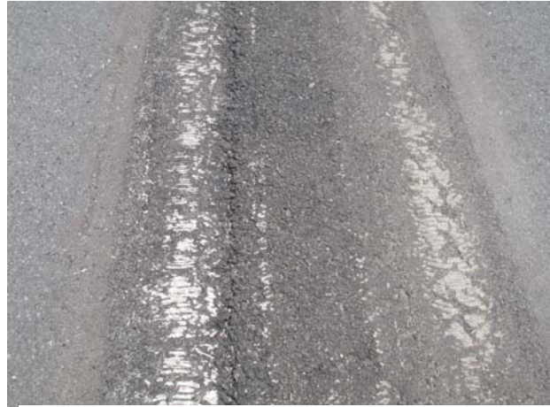
FIGURE 5-30. REMOVAL OF MULTIPLE LAYERS ON DETERIORATED ASPHALT.
