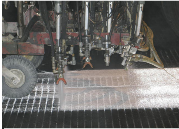
FIGURE 6-21. AIRLESS PAINT GUNS AND BEAD GUNS APPLYING MATERIAL TO PAVEMENT.
