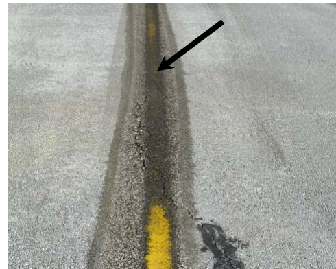
FIGURE 5-26. THE SCAR IS THE DARK PORTION OF THE ASPHALT THAT WAS SHIELDED FROM UV.
