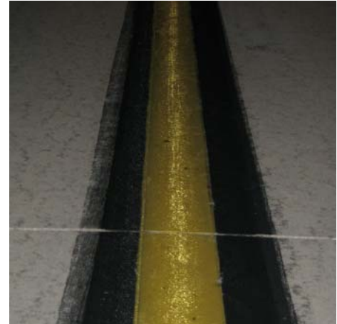
FIGURE 3-9. NON-FUNCTIONAL MARKING DUE TO POOR REFLECTIVITY.
