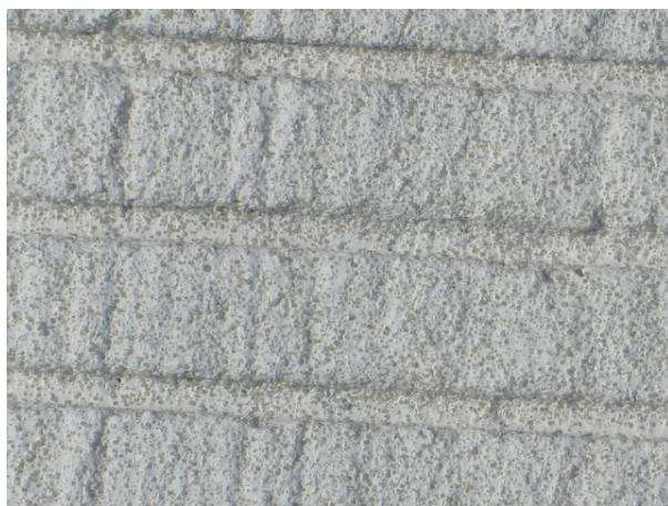
FIGURE 6-5. THE UNPAINTED SIDE OF THE GROOVES IS NOT NOTICEABLE FROM A DISTANCE.
