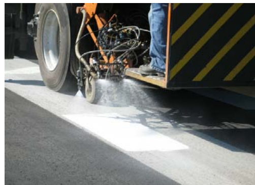
FIGURE 6-47. GLASS BEAD DISPENSERS ADJUSTED TOO HIGH.
