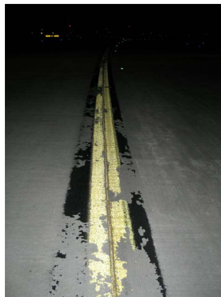
FIGURE 4-8. EXAMPLE OF POOR REMOVAL OF CURING COMPOUND.
