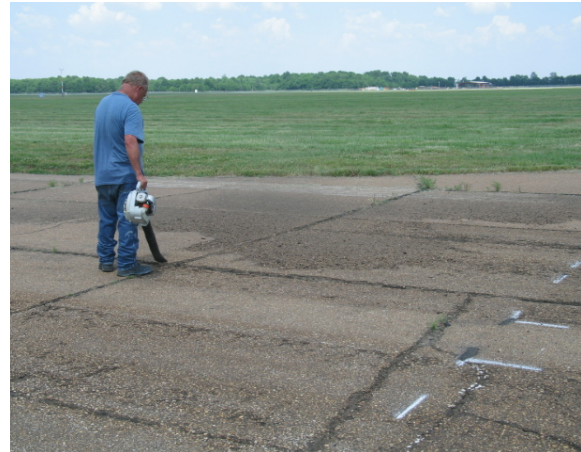
FIGURE 4-39. LEAF BLOWER CLEANS LOOSE RESIDUE AFTER SURFACE PREPARATION.
