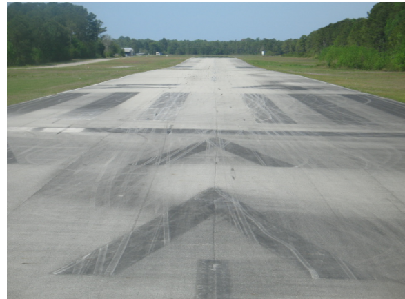
FIGURE 4-13. MARKINGS ARE OBSCURED BY ALGAE.
