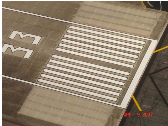
FIGURE 5-33. THE VISIBLE SCAR IS CLEANED PAVEMENT.
