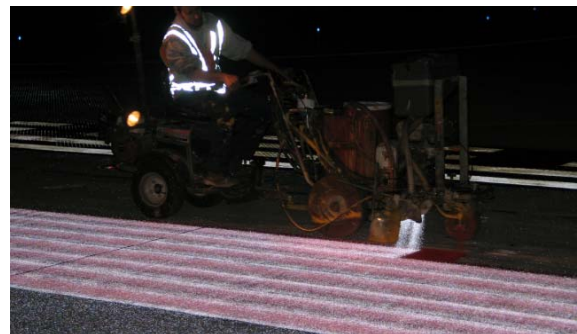
FIGURE 6-39. AN AIRLESS MACHINE WITH A MOTORIZED “SULKY” APPLIES MARKING WITH AUTOMATIC GLASS BEAD GUNS.
