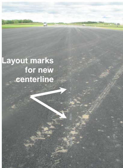
FIGURE 6-2. CONSTRUCTION DIRT MUST BE CLEANED.
