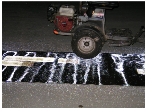
FIGURE 6-58 TEST LINES ON TAR PAPER.
