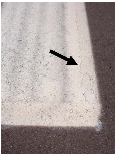
FIGURE 4-11. PAINT CRACKS WHEN APPLIED TOO THICKLY.
