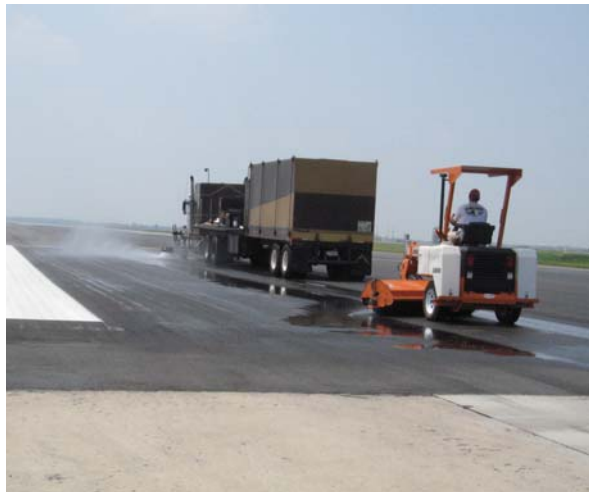
FIGURE 5-31. CLEANING THE REMOVAL SCAR BEFORE APPLICATION OF NEW MARKINGS.
