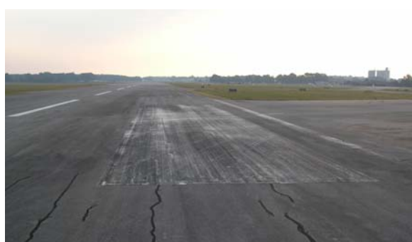
FIGURE 4-16. BEFORE WATERBLASTING: ALGAE OBSCURE MARKING.
