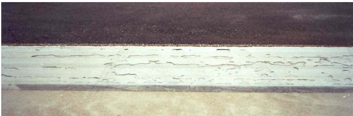
FIGURE 4-3. REPEATED PAINTING ON CONCRETE LEADS TO FOD.
