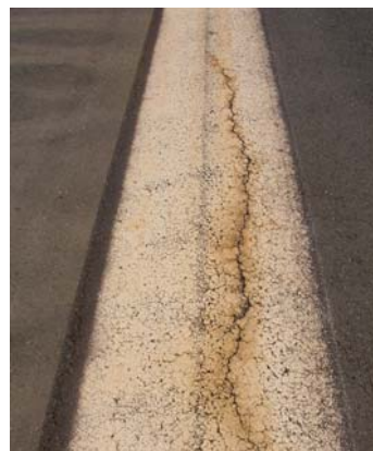
FIGURE 4-27. EVIDENCE OF RUST CONTAMINATION FROM SUBSTRATE.
