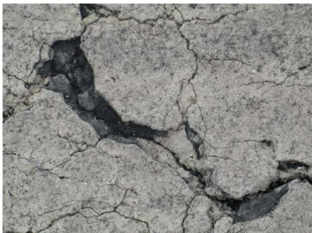
FIGURE 5-29. CRACKED PAINT INDICATES PRE-EXISTING PAVEMENT DETERIORATION.
