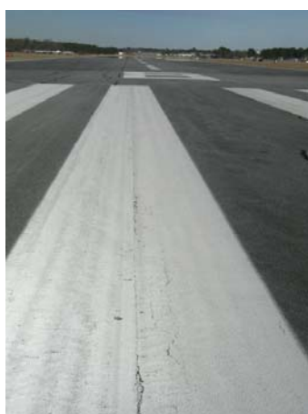
FIGURE 4-19. PAINT FORMULATED TO RESIST ALGAE.
