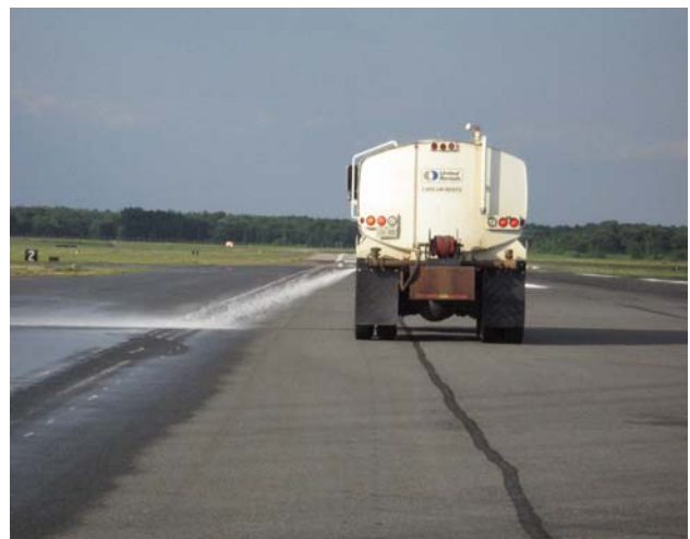
FIGURE 5-32. A BLAST OF HIGH-PRESSURE WATER REMOVES DEBRIS FROM SCAR.
