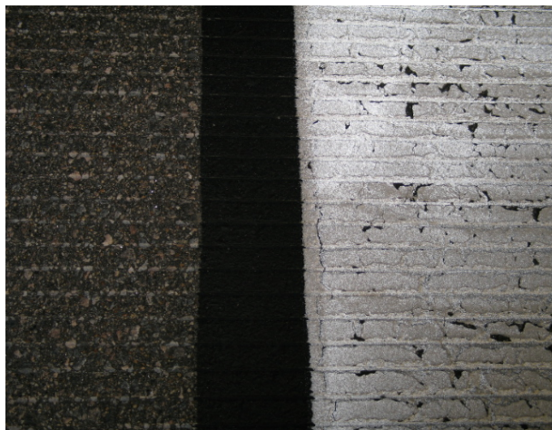
FIGURE 5-10. BEFORE PAINT REMOVAL.
