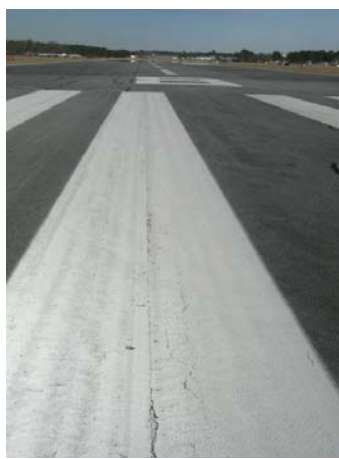
FIGURE 4-19. PAINT FORMULATED TO RESIST ALGAE.
