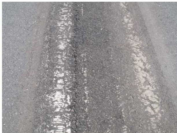
FIGURE 5-30. REMOVAL OF MULTIPLE LAYERS ON DETERIORATED ASPHALT.
