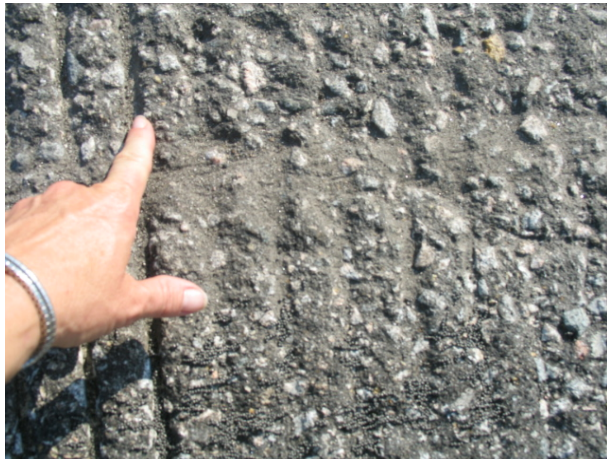
FIGURE 5-12. AFTER REMOVAL OF THE MARKINGS ON GROOVED PAVEMENT WITH SHOTBLASTING.
