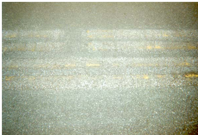
FIGURE 5-8. MINIMAL GRINDER SCARS ON ASPHALT AFTER REMOVING 90 PERCENT.
