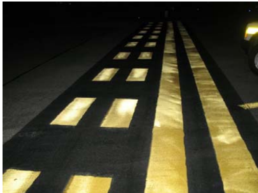
FIGURE 6-34. NEW HOLDING POSITION MARKING WHERE BEADS WERE HAND-THROWN.
