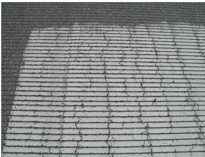
FIGURE 4-12. PAINT BONDS BETTER TO ASPHALT THAN ASPHALT DOES TO ITSELF.
