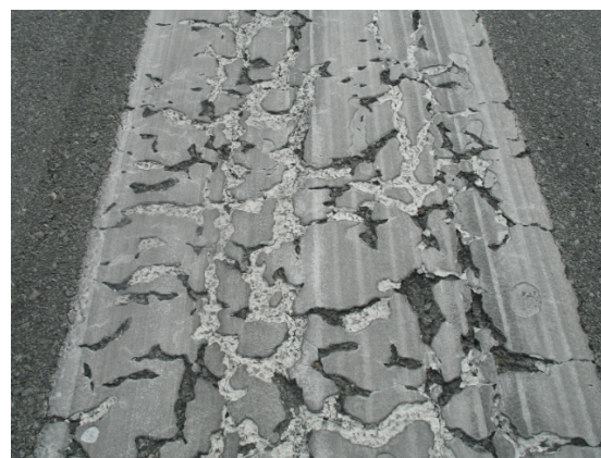
FIGURE 4-7. MANY LAYERS OF PAINT ON ASPHALT.
