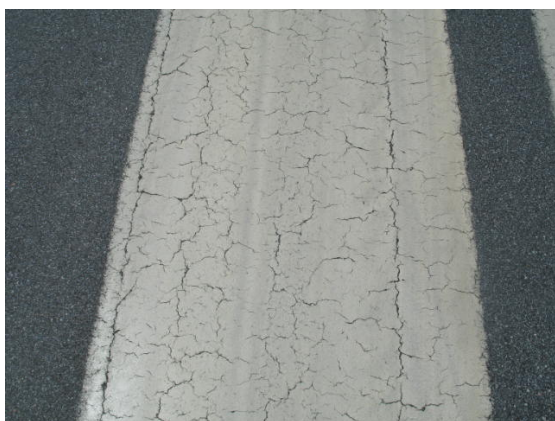
FIGURE 4-6. THIS MARKING IS 30 MONTHS OLD AND CRACKED.
