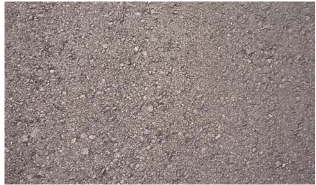
FIGURE 4-10. AFTER RUBBER REMOVAL.
