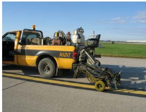
FIGURE 6-22. SKID MOUNTED PAINT RIG APPLIED BLACK BACKGROUND FOR TAXIWAY CENTERLINE IN FIGURE 6-23.
