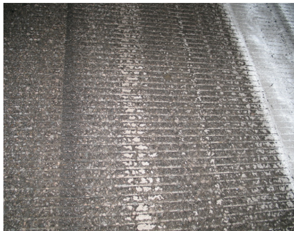
FIGURE 5-11. AFTER PAINT REMOVAL WITH A SHOTBLASTER ON GROOVED ASPHALT.
