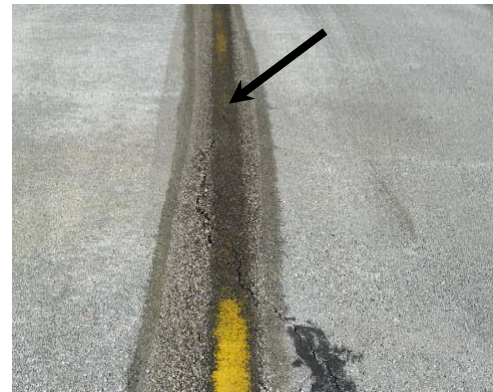
FIGURE 5-26. THE SCAR IS THE DARK PORTION OF THE ASPHALT THAT WAS SHIELDED FROM UV.
