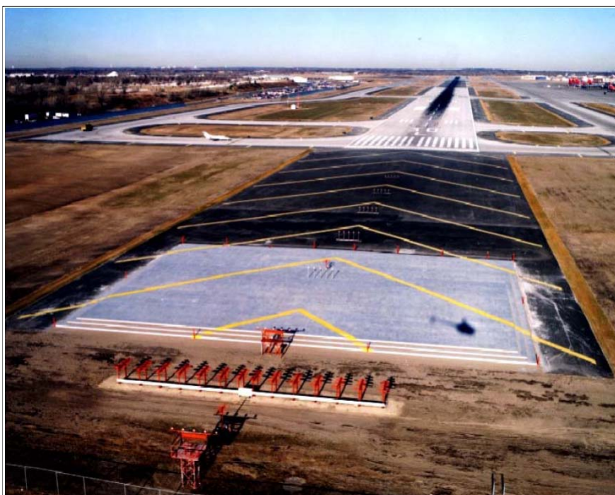
FIG 2-3-42 Engineered Materials Arresting System (EMAS)
