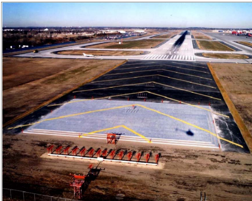
FIG 2-3-42 Engineered Materials Arresting System (EMAS)
