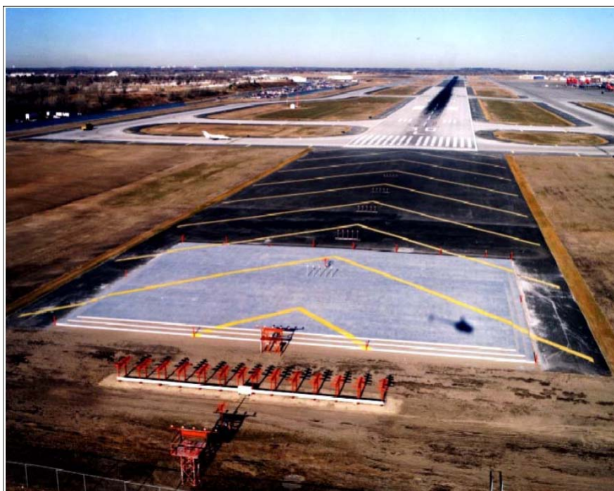
FIG 2-3-42 Engineered Materials Arresting System (EMAS)
