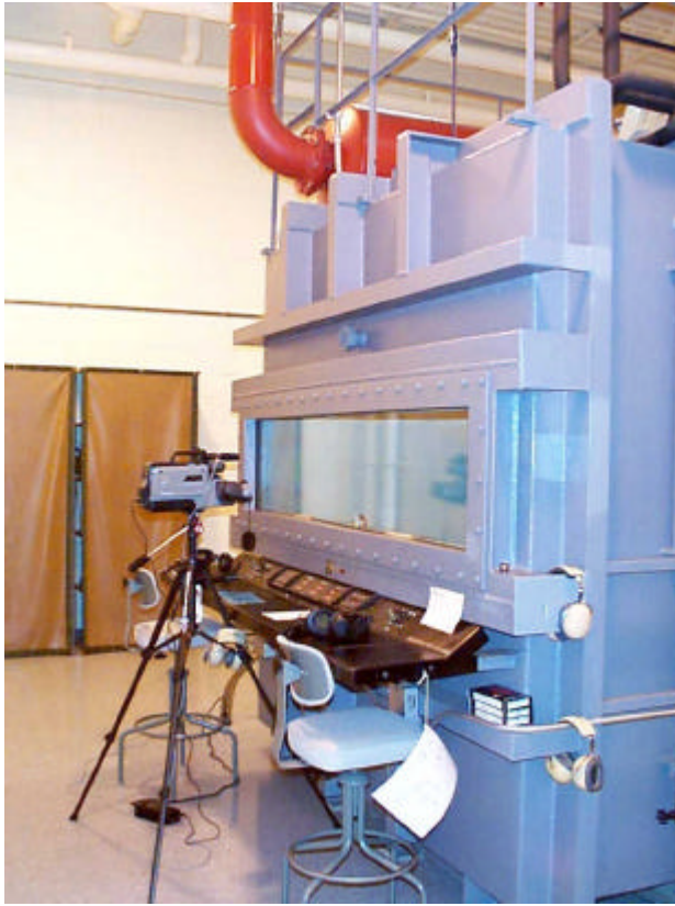
PHOTO 4 Decompression Chamber - Front Elevation
