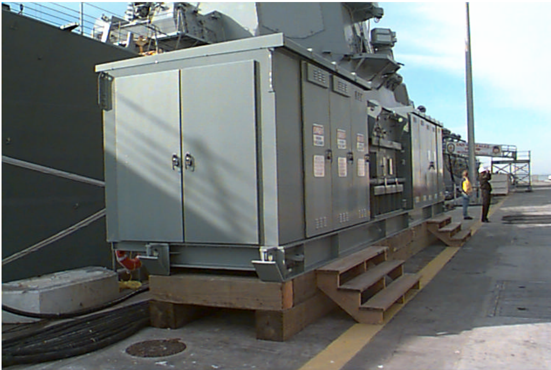
Picture C. A skid-mounted substation
