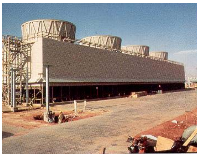
Figure 4-9. Counter-Flow Cooling Tower
