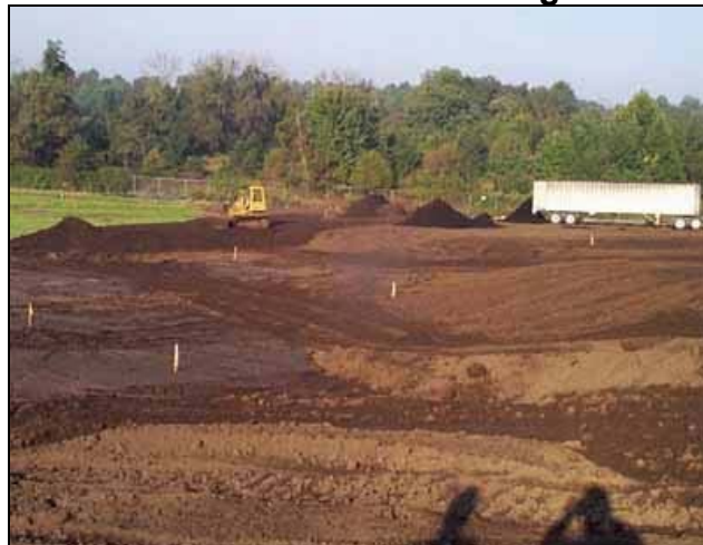
Figure 8-1. Southern Maryland Wood Treating Site: On-site Thermal Desorption of Contaminated Soils. Final Grading and LeafGro® Placement
