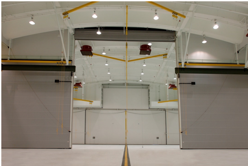
Figure E-14: Vertical Lift Fabric Door Mullion and Mullion Pit
