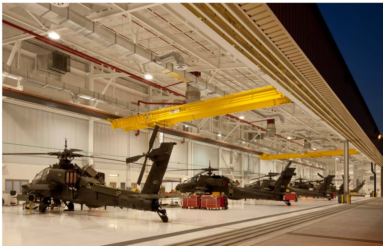
Figure E-6: Helicopter Hangar Bay with Sliding Doors, Sliding Door Tracks and Overhead Cranes
