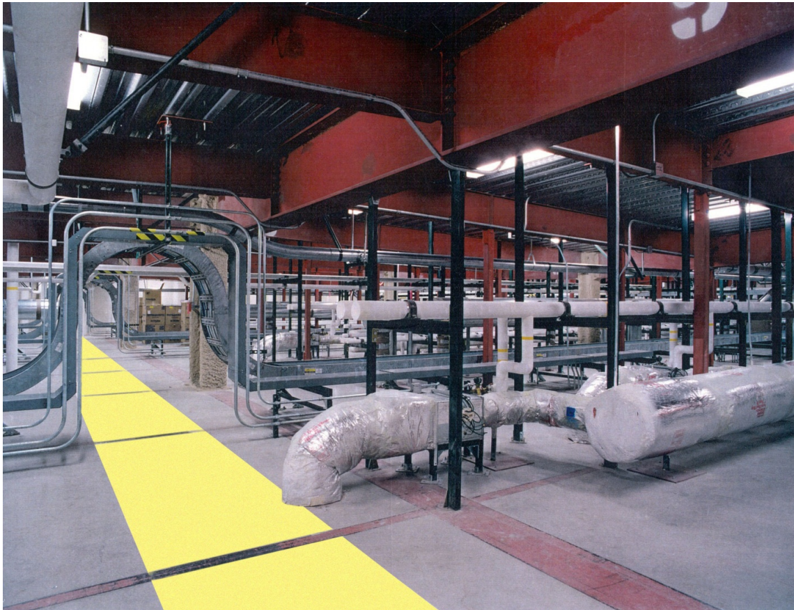
Figure E-3 Interstitial Access-Egress (Typical)
