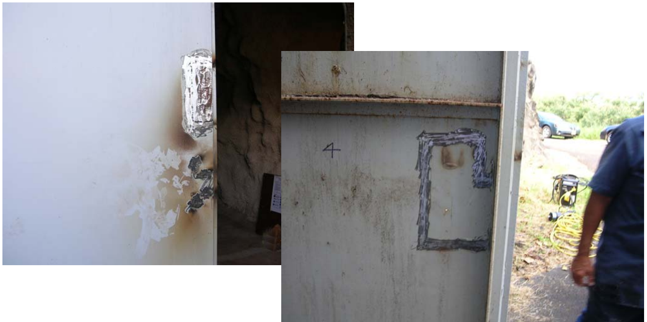
Figure B-7. Tack weld the boltwork housing assembly
