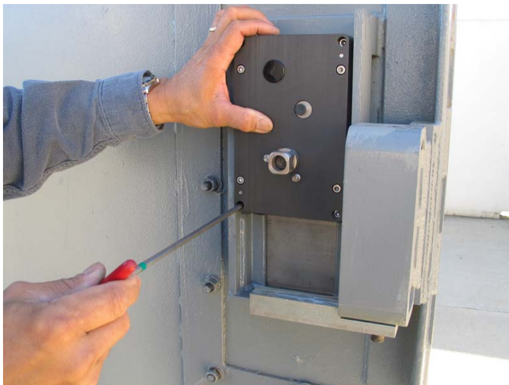
Figure D-5. Removal of ILD mounting screws
