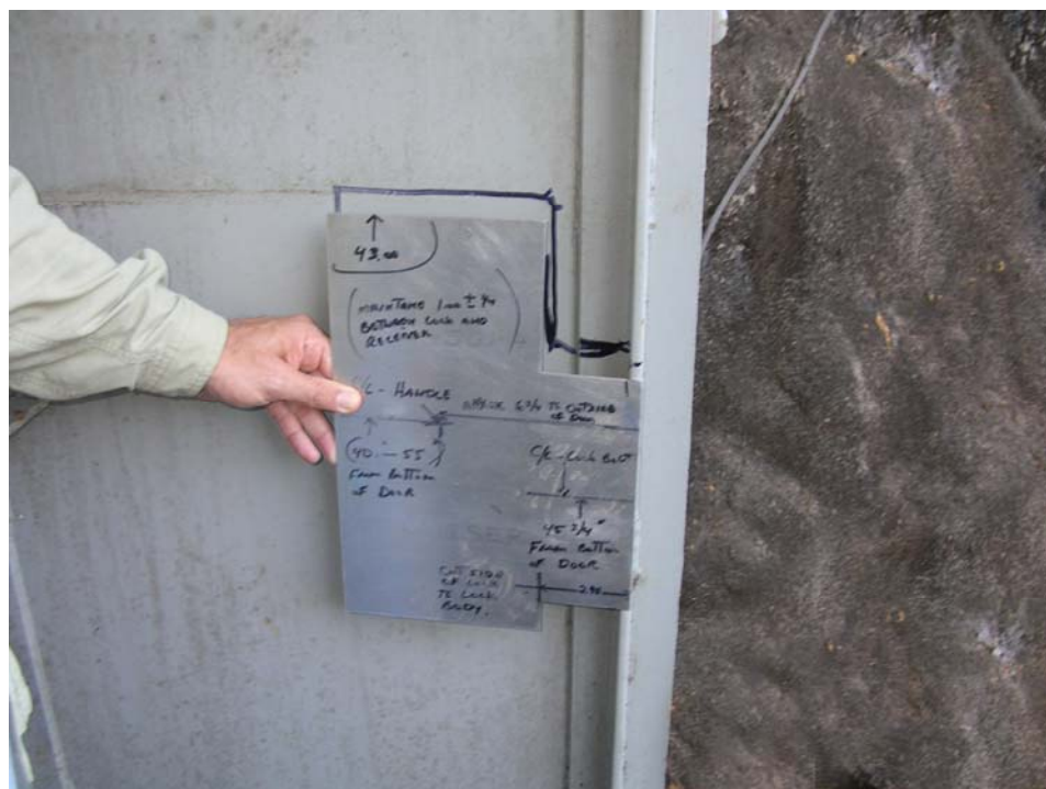
Figure B-5. Locate the ILD on the door
