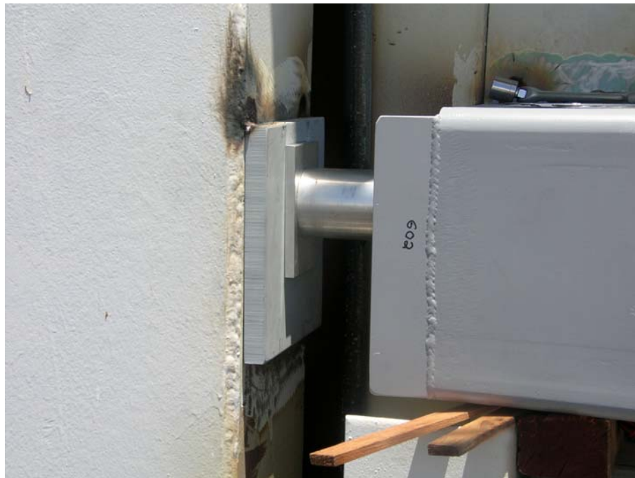
Figure C-12. Tack weld the receiver plate to the magazine door
