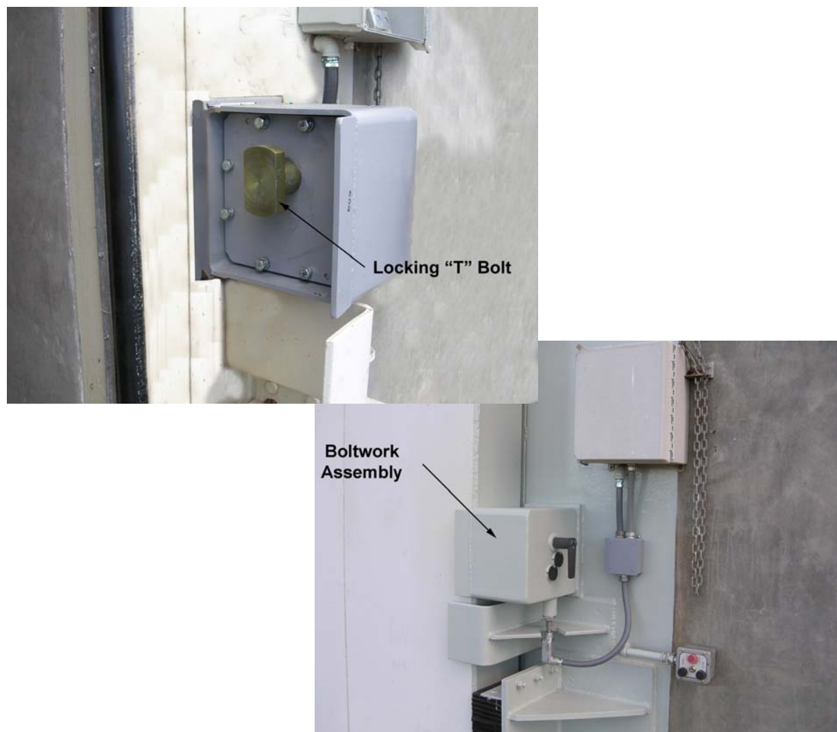
Figure 2-6. Locking “T” bolt and boltwork assembly for sliding magazine doors
