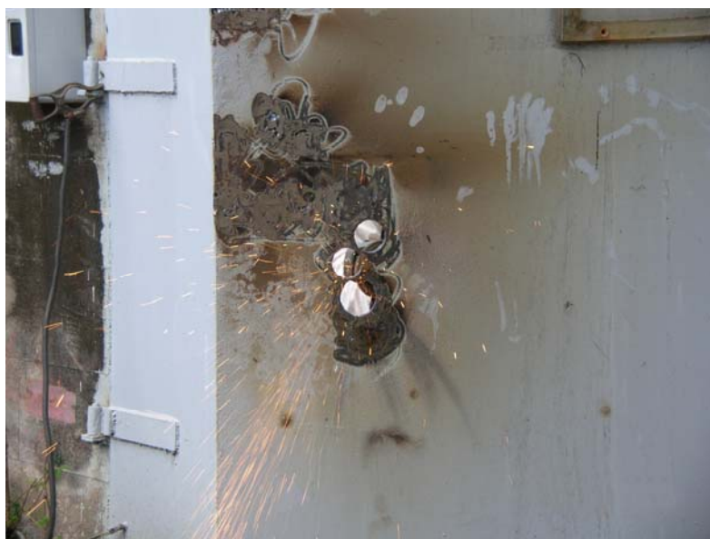
Figure B-9. Drill holes for handle and key guide bushings using hole saws or a plasma cutter
