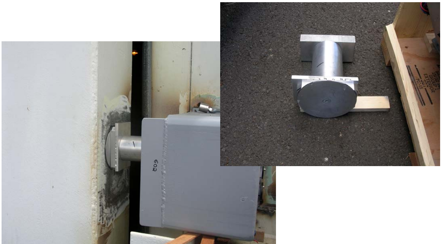
Figure C-8. Locate the receiver plate position using the "T" bolt alignment tool
