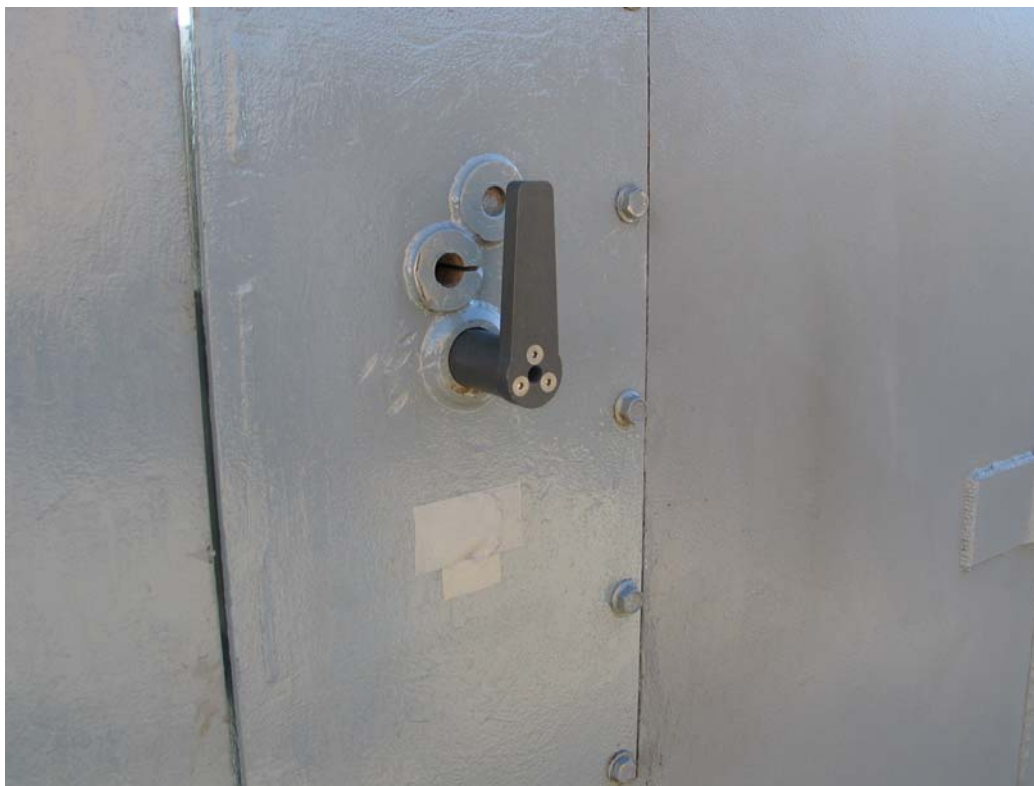
Figure D-4. Removal of ILD lever arm (handle)
