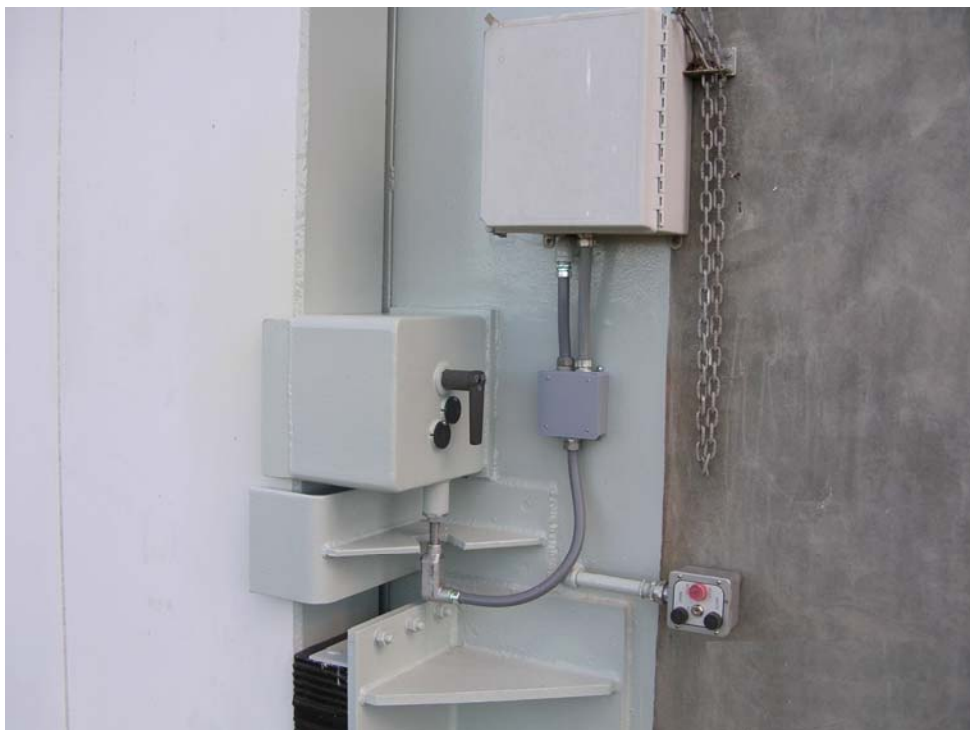
Figure C-14. Paint bare metal surfaces to protect against corrosion
