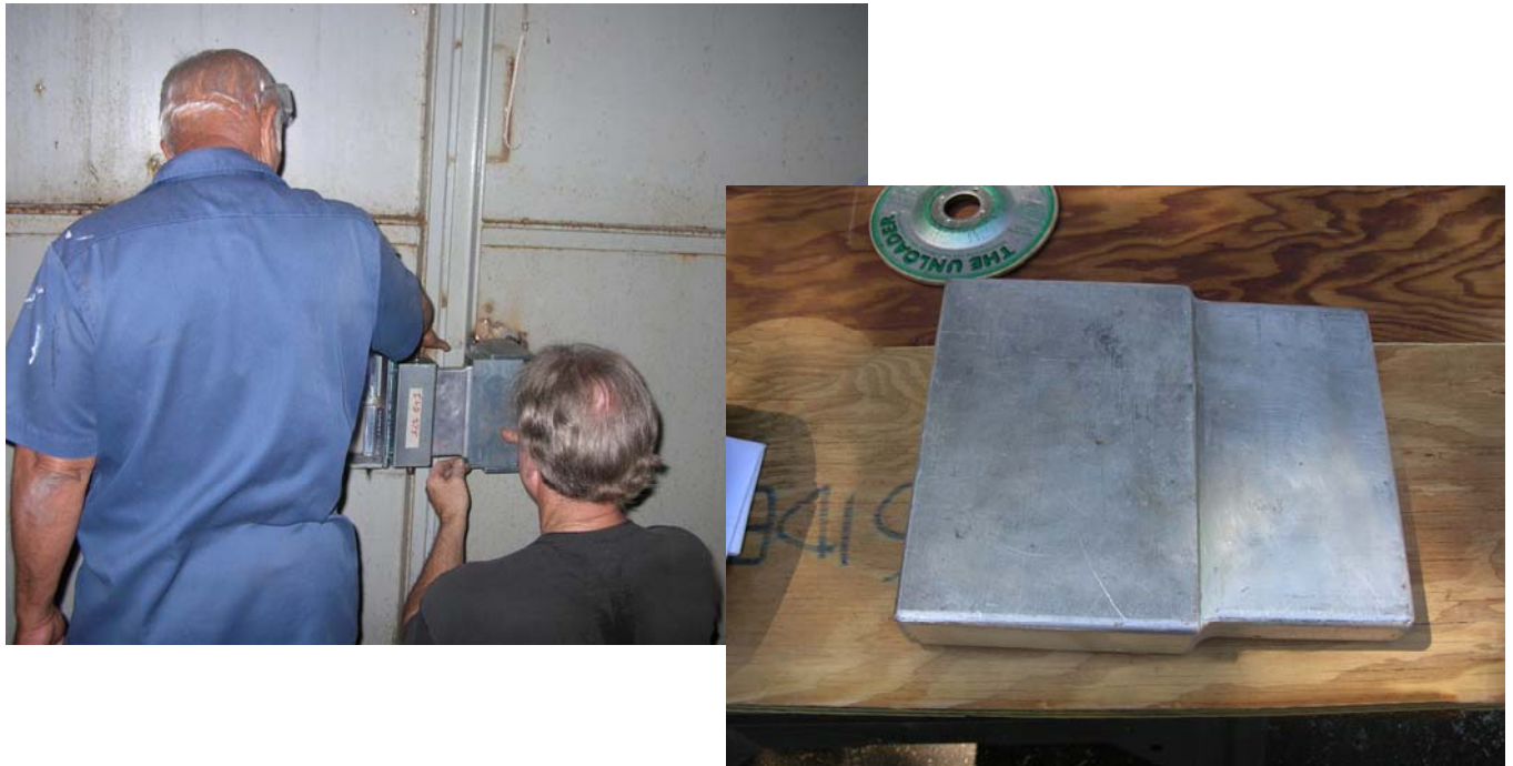
Figure B-12. Use receiver alignment tool to properly align retaining tube with boltwork assembly
