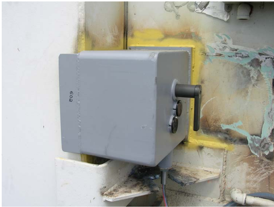
Figure C-14. Paint bare metal surfaces to protect against corrosion
