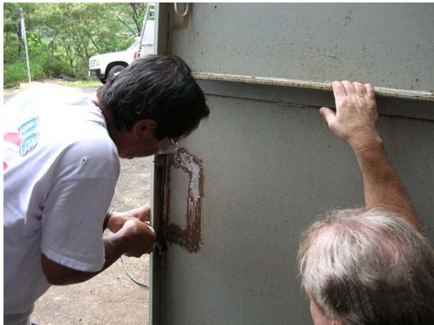
Figure B-11. Prepare surface for welding retaining tube bracket
