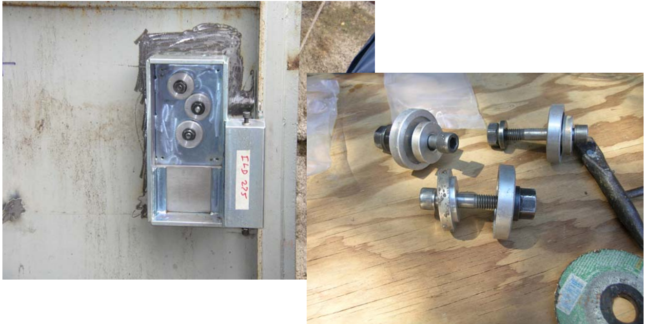
Figure B-11. Prepare surface for welding retaining tube bracket
