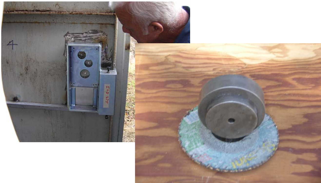
Figure B-9. Drill holes for handle and key guide bushings using hole saws or a plasma cutter
