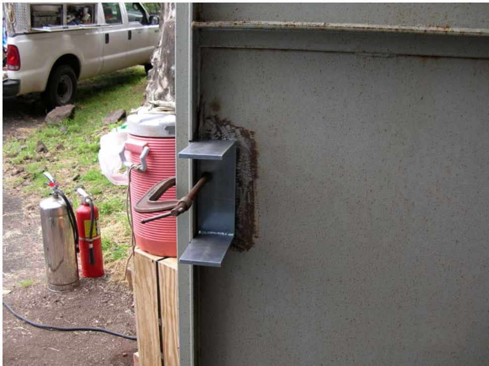
Figure B-13. Install the retaining tube bracket on inactive door
