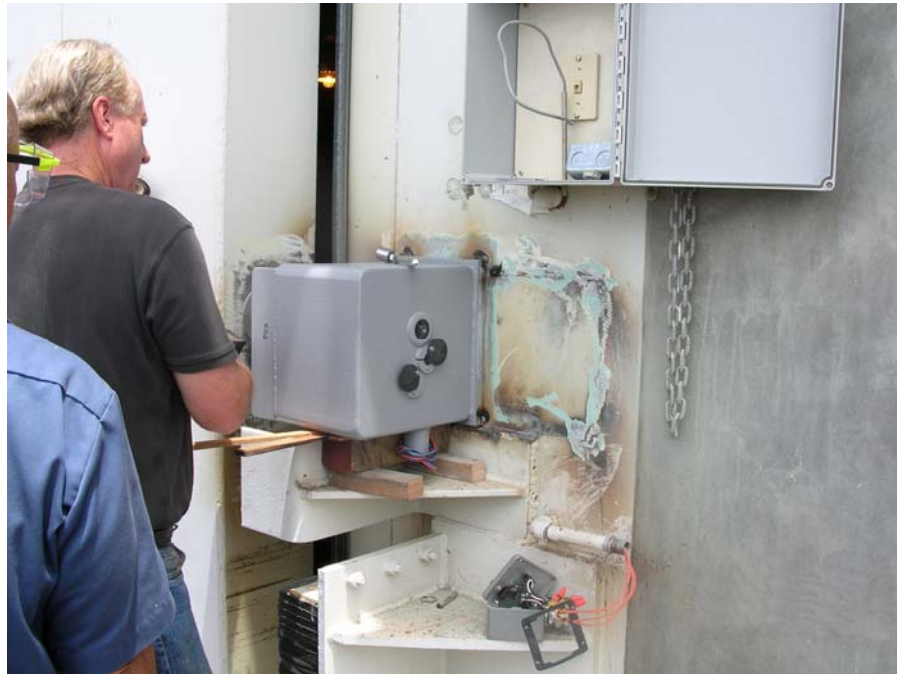
Figure C-8. Locate the receiver plate position using the "T" bolt alignment tool
