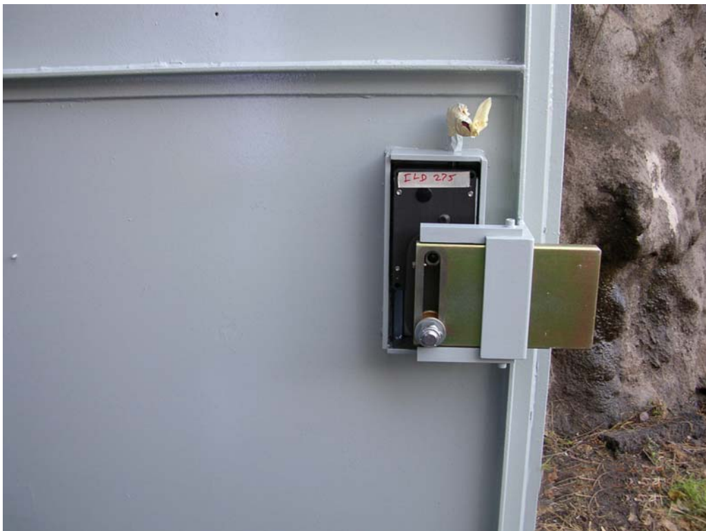
Figure D-8. Reassembled swinging door boltwork
