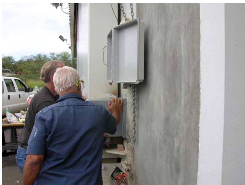
Figure C-6. Position the ILD boltwork assembly on the headwall
