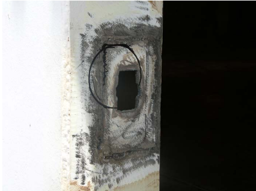
Figure C-10. Cut circular hole to receive the “T” bolt
