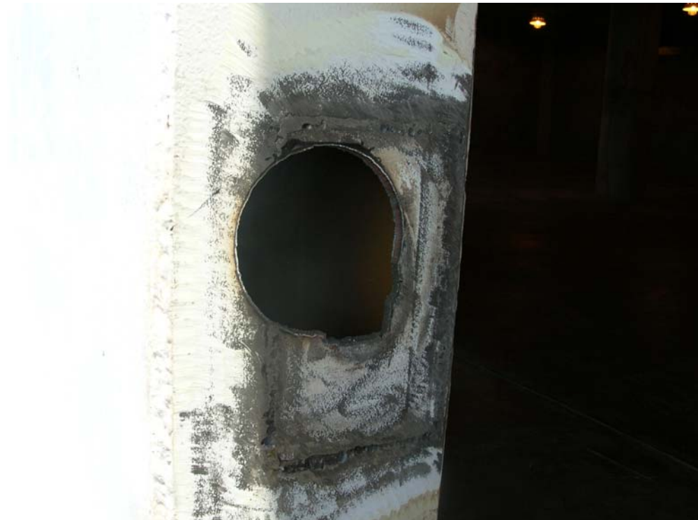
Figure C-10. Cut circular hole to receive the “T” bolt
