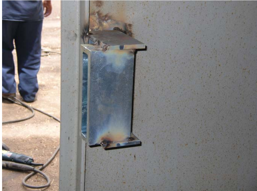
Figure B-15. Weld all assemblies in place
