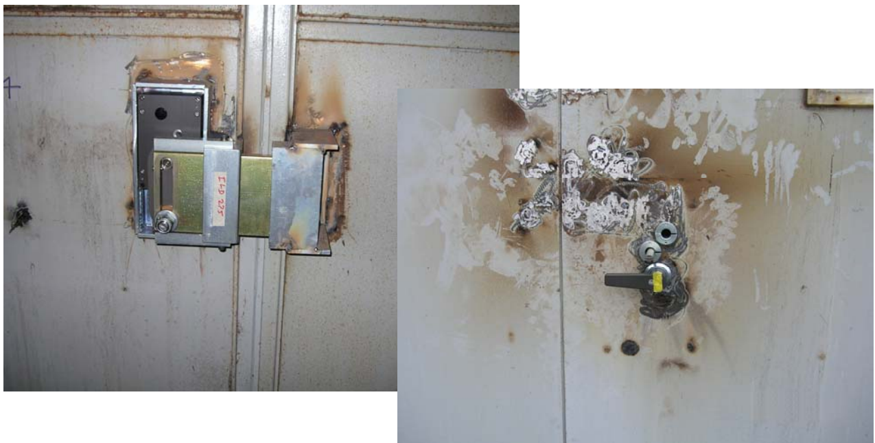
Figure B-15. Weld all assemblies in place
