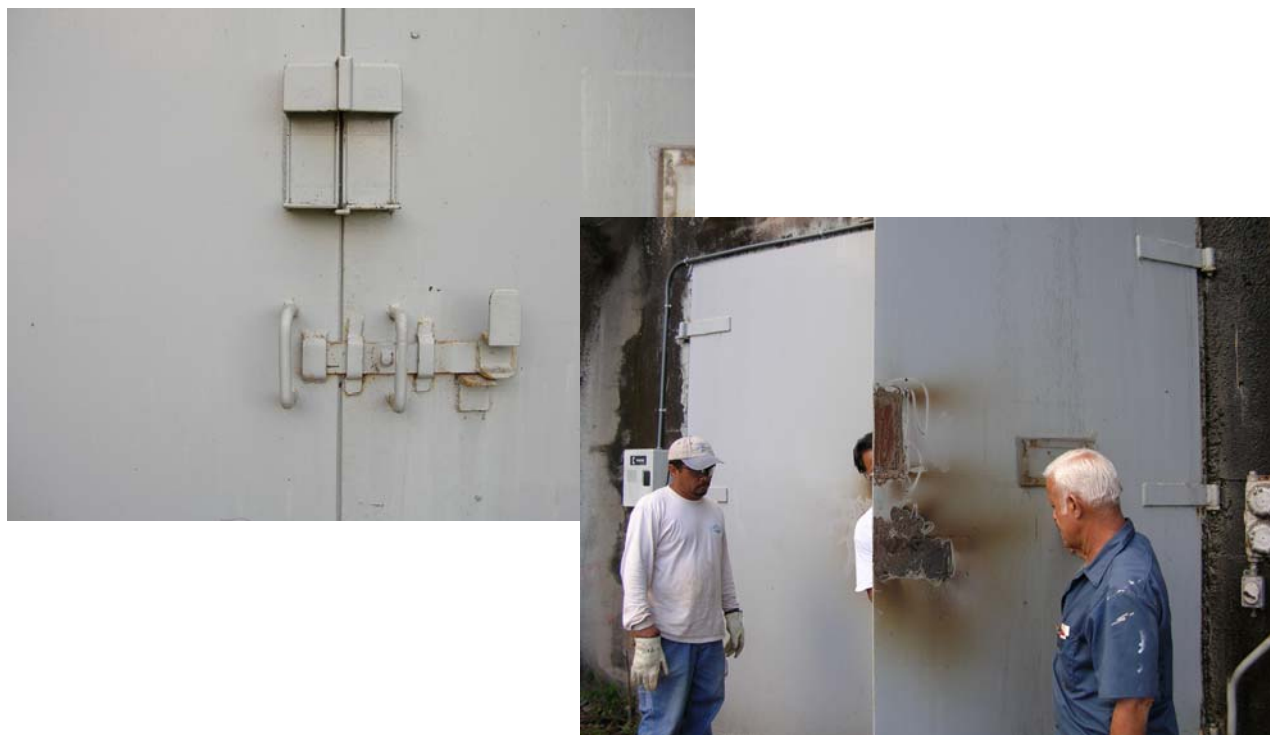
Figure B-4. Remove obstructions from the door
