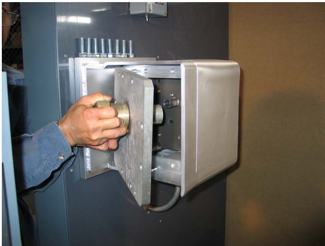
Figure D-9. Removal of bolts and boltplate
