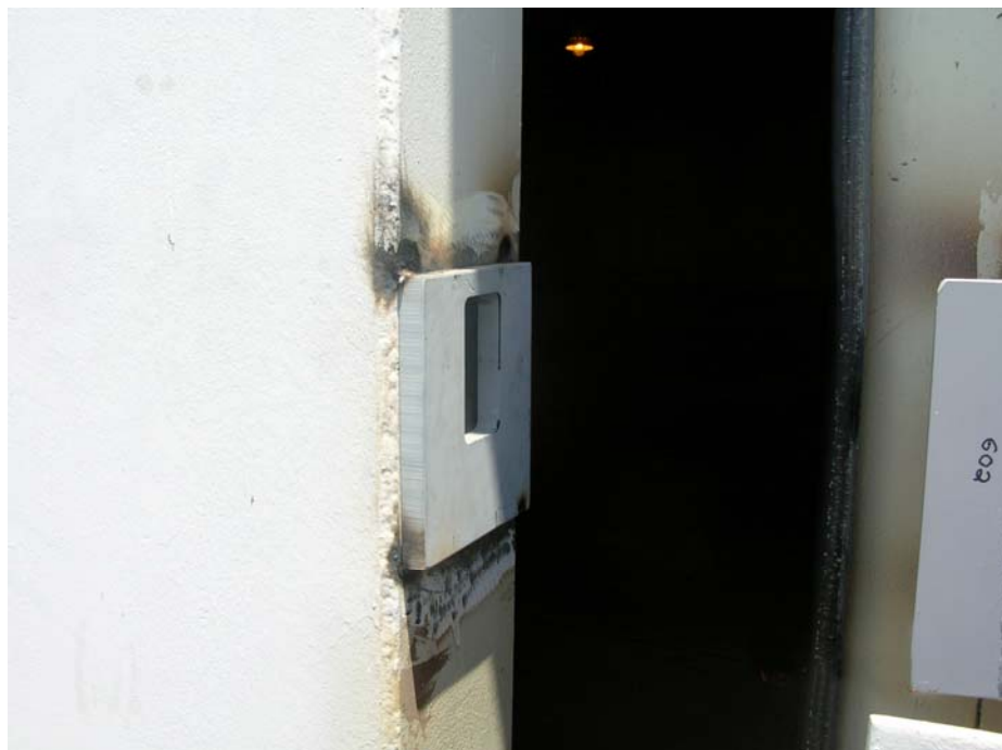
Figure C-12. Tack weld the receiver plate to the magazine door
