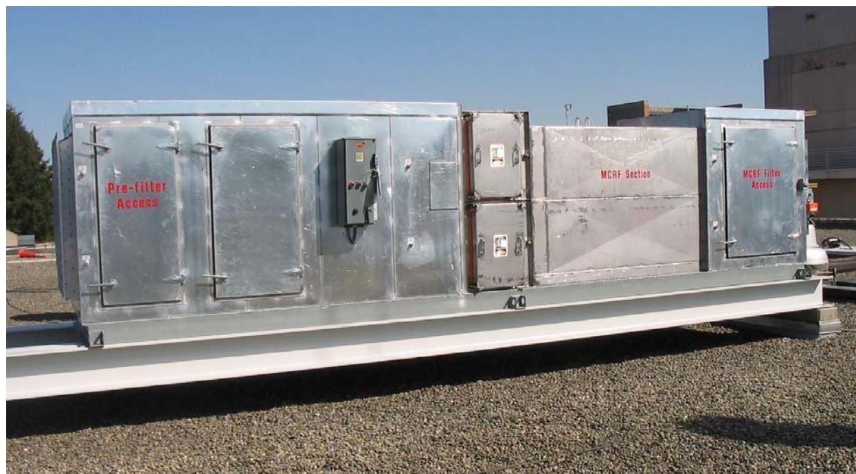
Figure G-12. Multi-Cell Radial-Flow (MCRF) Filtration Unit
