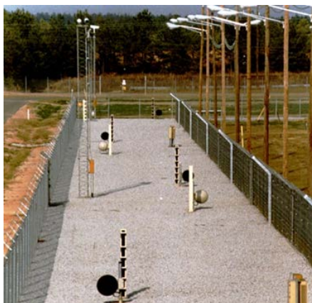
Figure 5-12. Double Fence Example.
