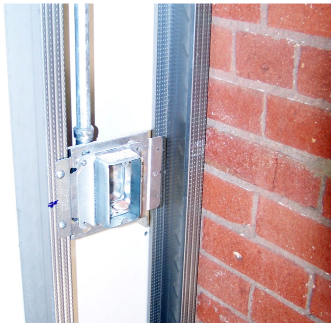
Figure 3-3 Furred Out Wall for Utilities
