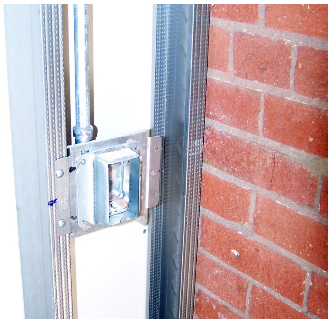
Figure 3-3 Furred Out Wall for Utilities
