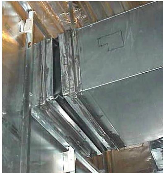
Figure 3-6 Duct Penetrations
