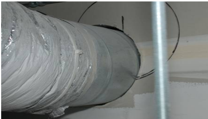
Figure 3-7 Sealing Penetrations
