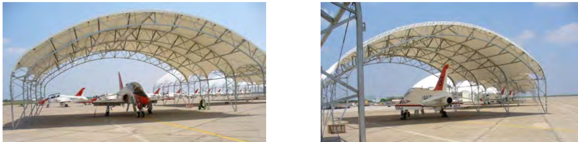
Figure 6-7 Examples of Weather Covering
