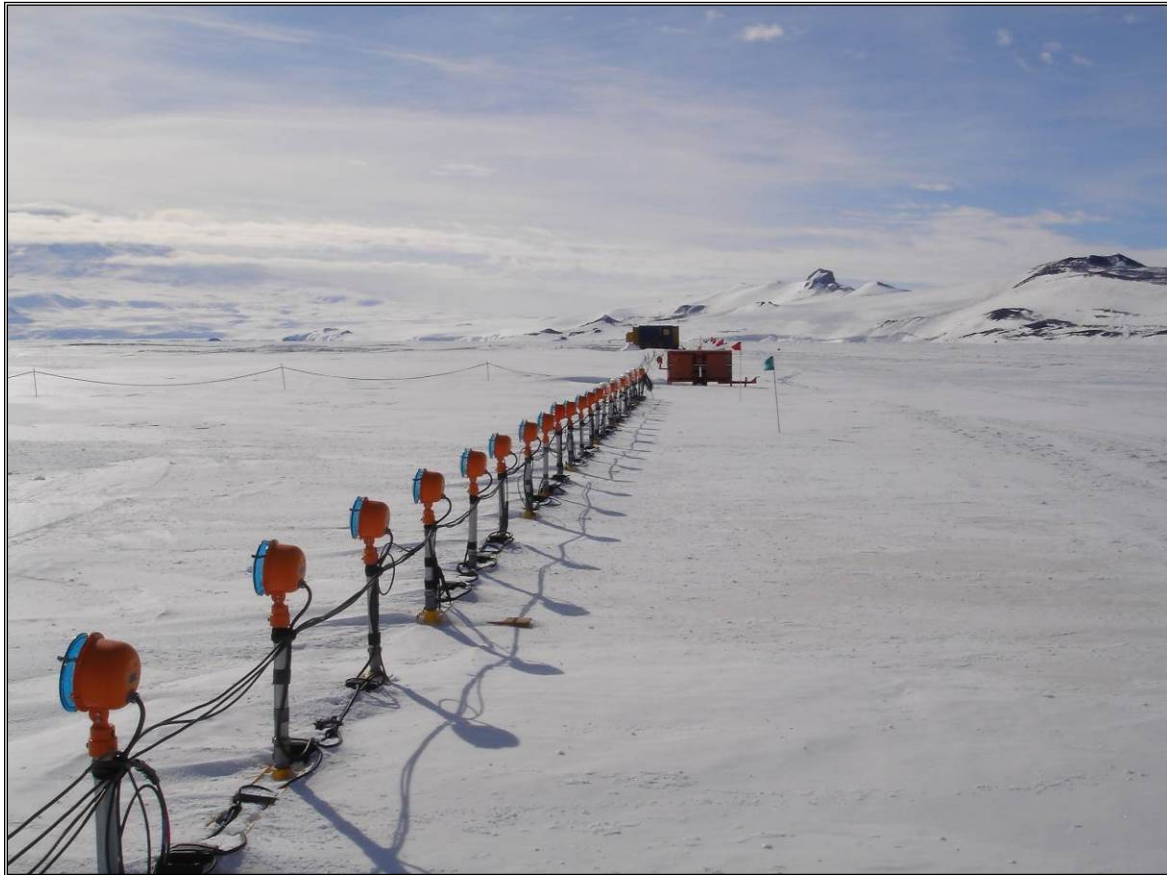
Figure 2-10 Typical Threshold Light Installation for Snow/Ice Airfields
