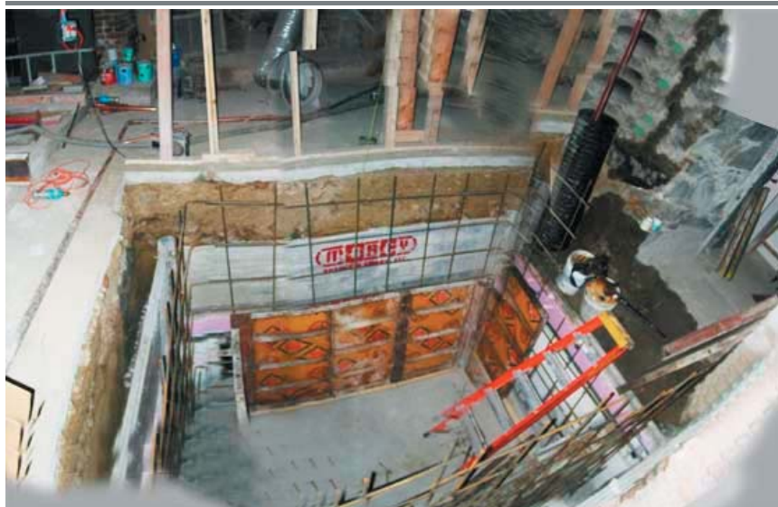
Construction of an elevator pit
