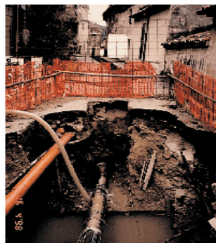
"Open cut", a well established technique.
