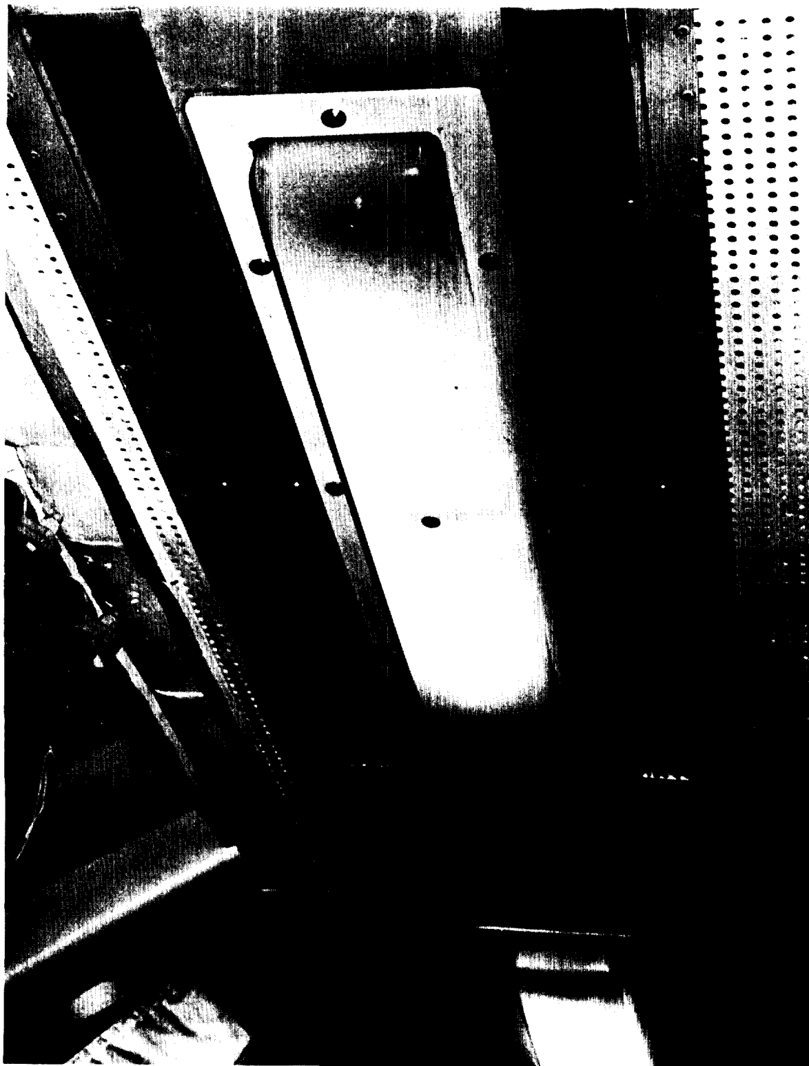
FIGURE 103. Typical flush mounting of fluorescent lighting fixtures. (For details see method E-1-B of appendix B)
