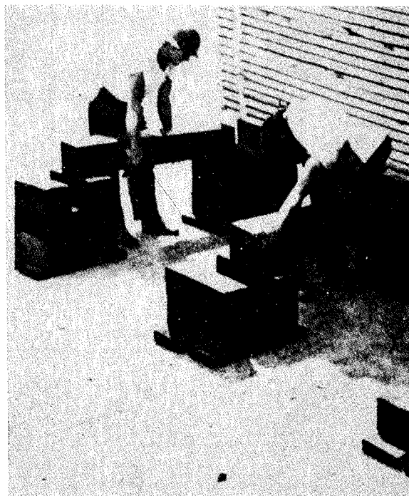
Figure 5-10. Application of the portable lumber foundation.
