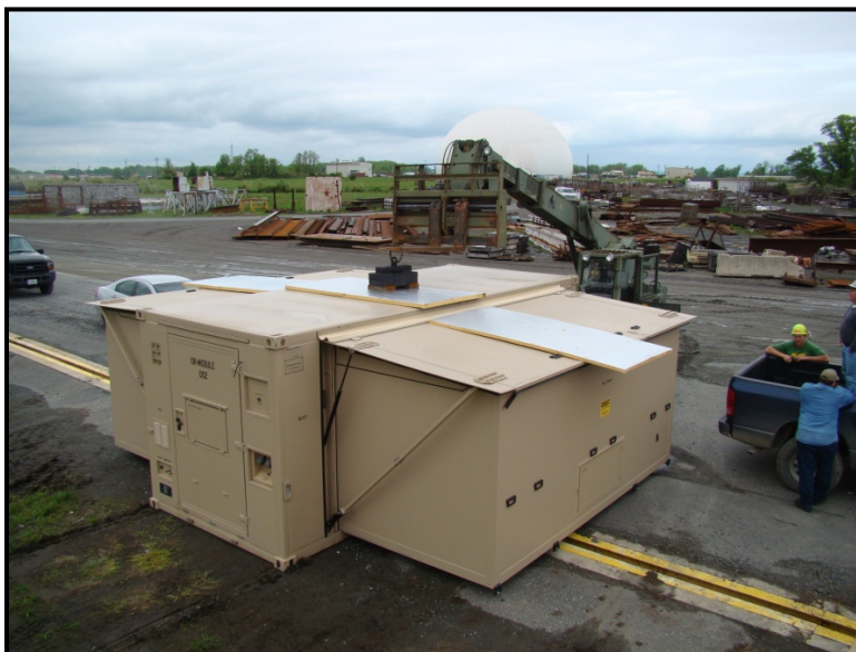
Figure 4. Two-sided medical operating room with rigid walls and expandable floors.
