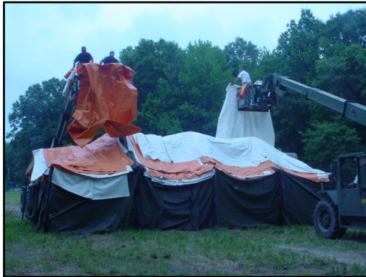
Figure 10. Snow load test of framed tent
