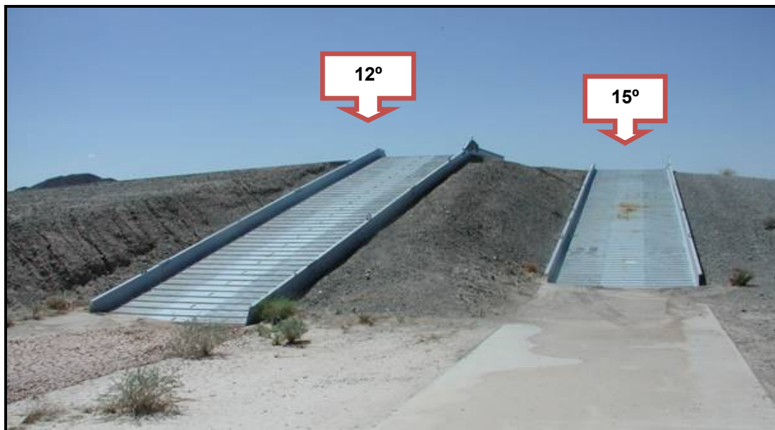
Figure 124. 12 degree roll on/roll off ramp (left) and 15 degree roll on/roll off ramp (right).
