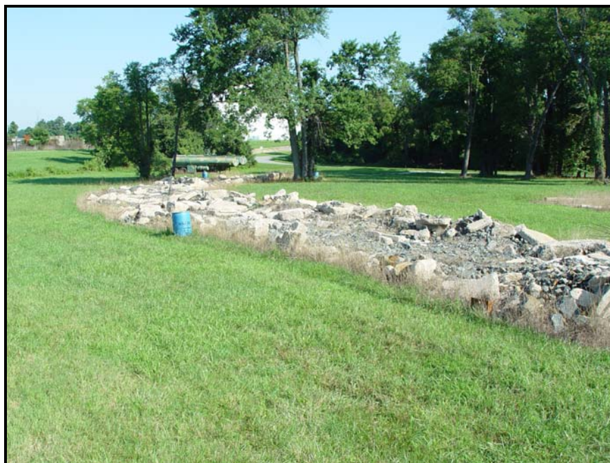
Figure 26. Rubble Pile at MTA.
