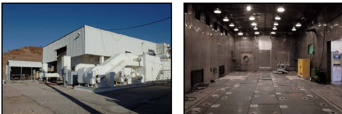
Figure 177. Outside view of LMPEC (left) and view into LMPEC from access door opening (right).
