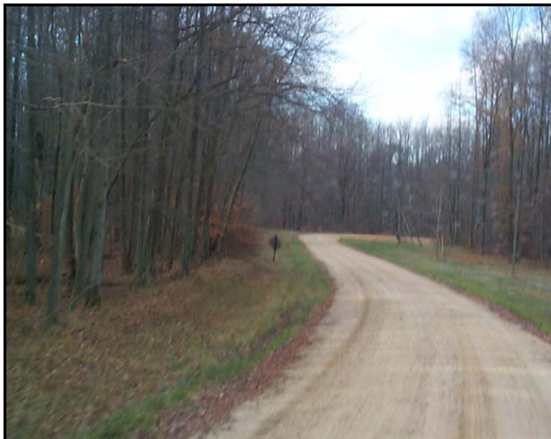
Figure 73. Perryman No. 1 roadbed characteristics.
