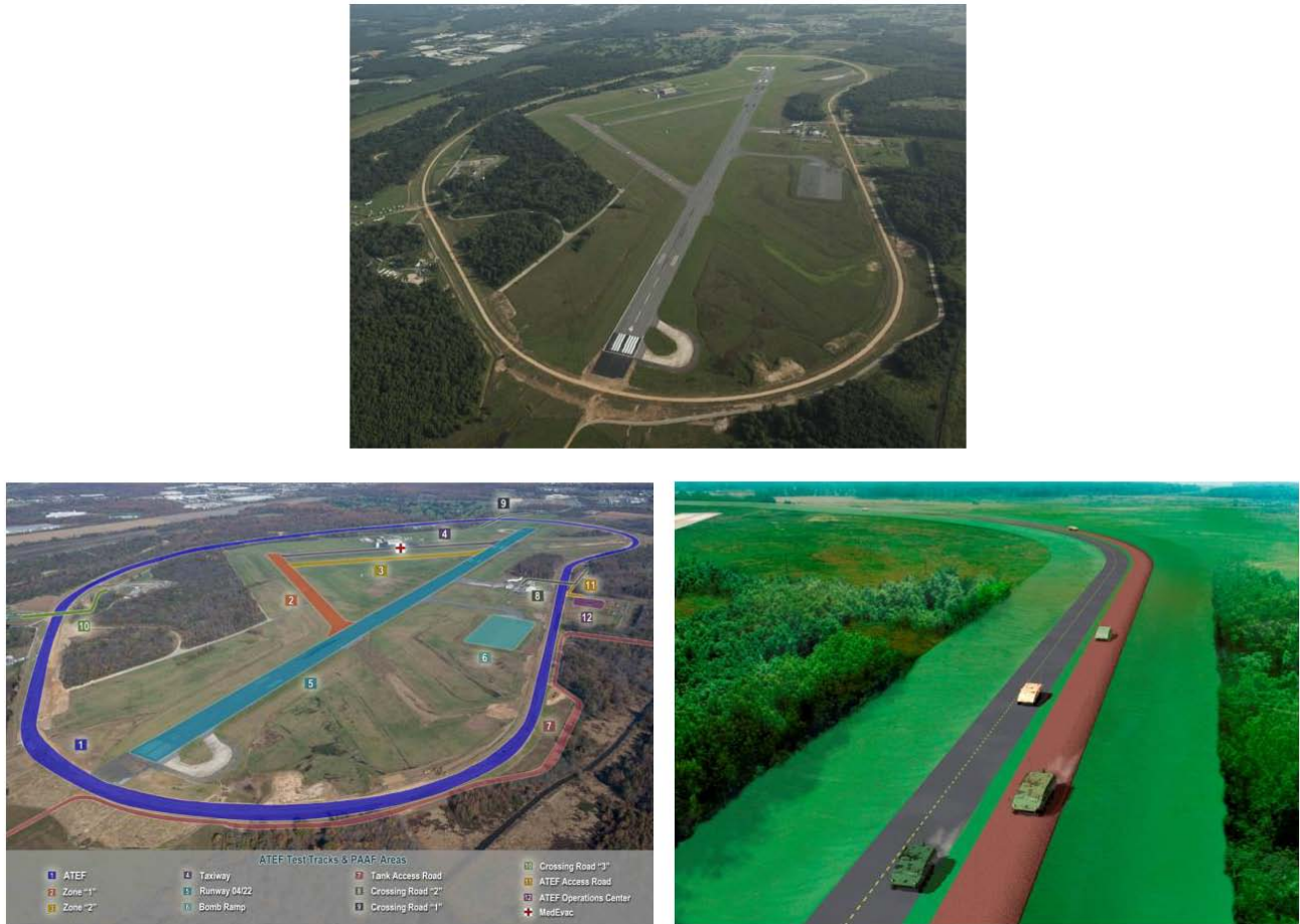
Figure 70. Automotive Technology Evaluation Facility.
