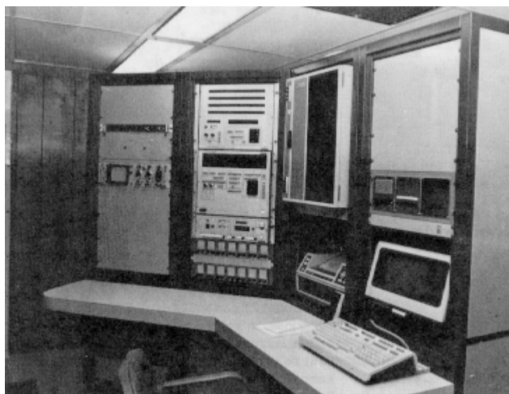
Figure 79. Test site terminal -interior view
