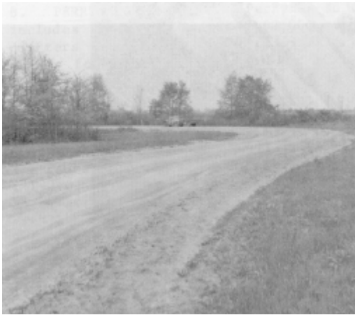
Figure 64. View of roadbed characteristics, cross-country course No.1.
