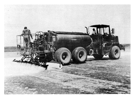
Figure 3-1. Special distributor for the three-step process of applying the DCA 1295.
