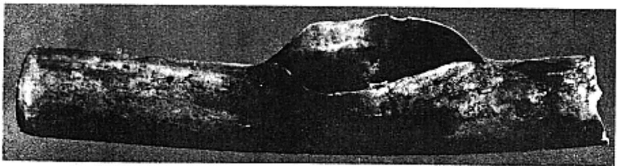
FIGURE 4-2. BOILER TUBE FAILURE CAUSED BY SCALE
