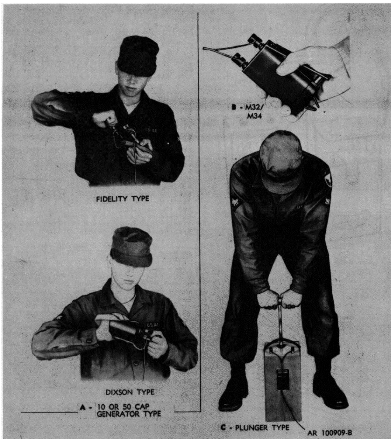
Figure 4-20. Actuating blasting machines.
