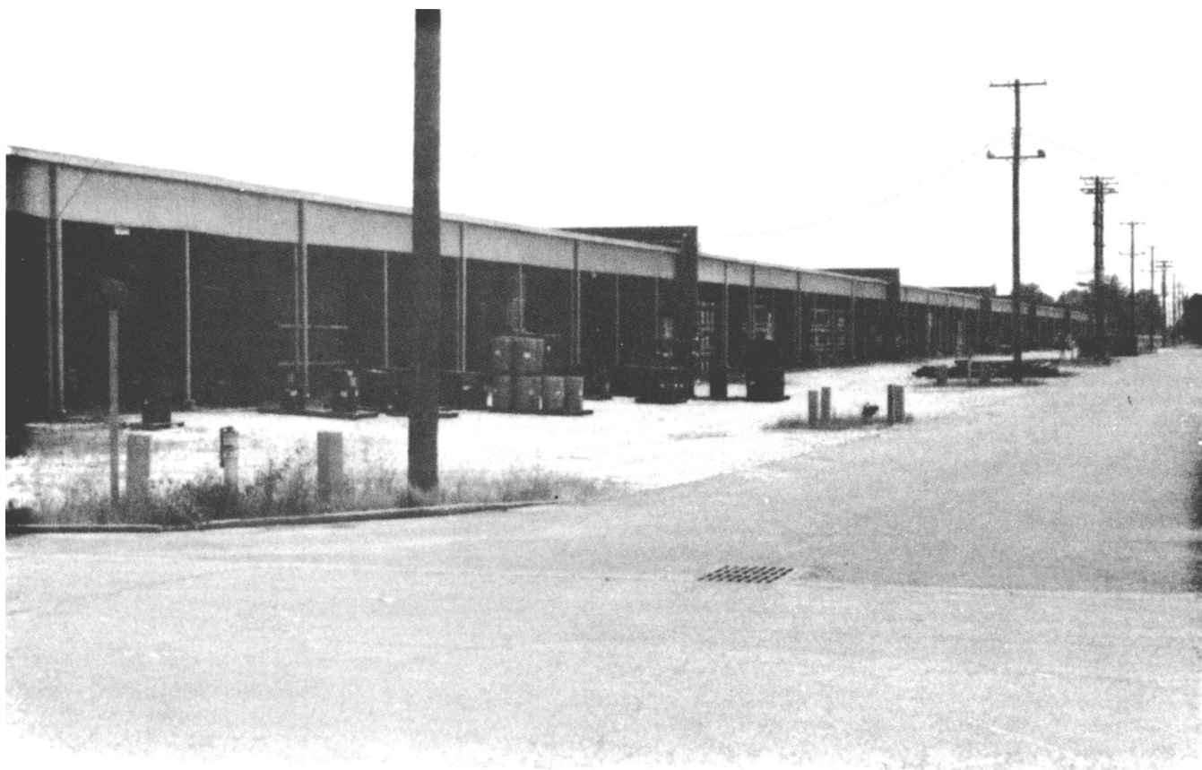
Figure 4-1. Storage shed with floor at road level.
