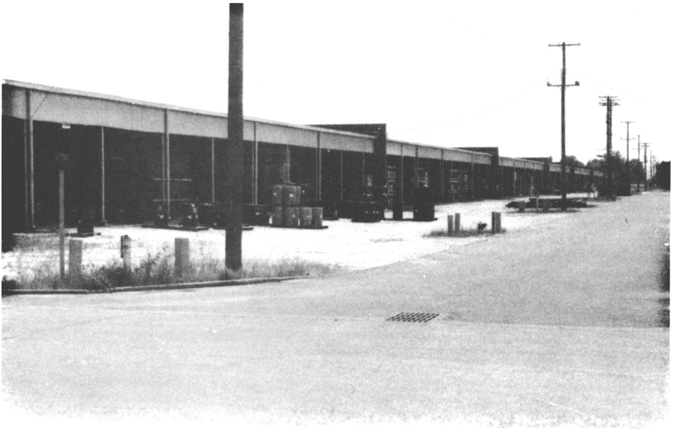
Figure 4-1. Storage shed with floor at road level.
