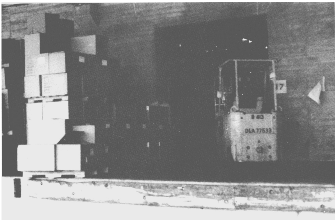
Figure 3-5. Loading dock showing wooden protective bumpers.
