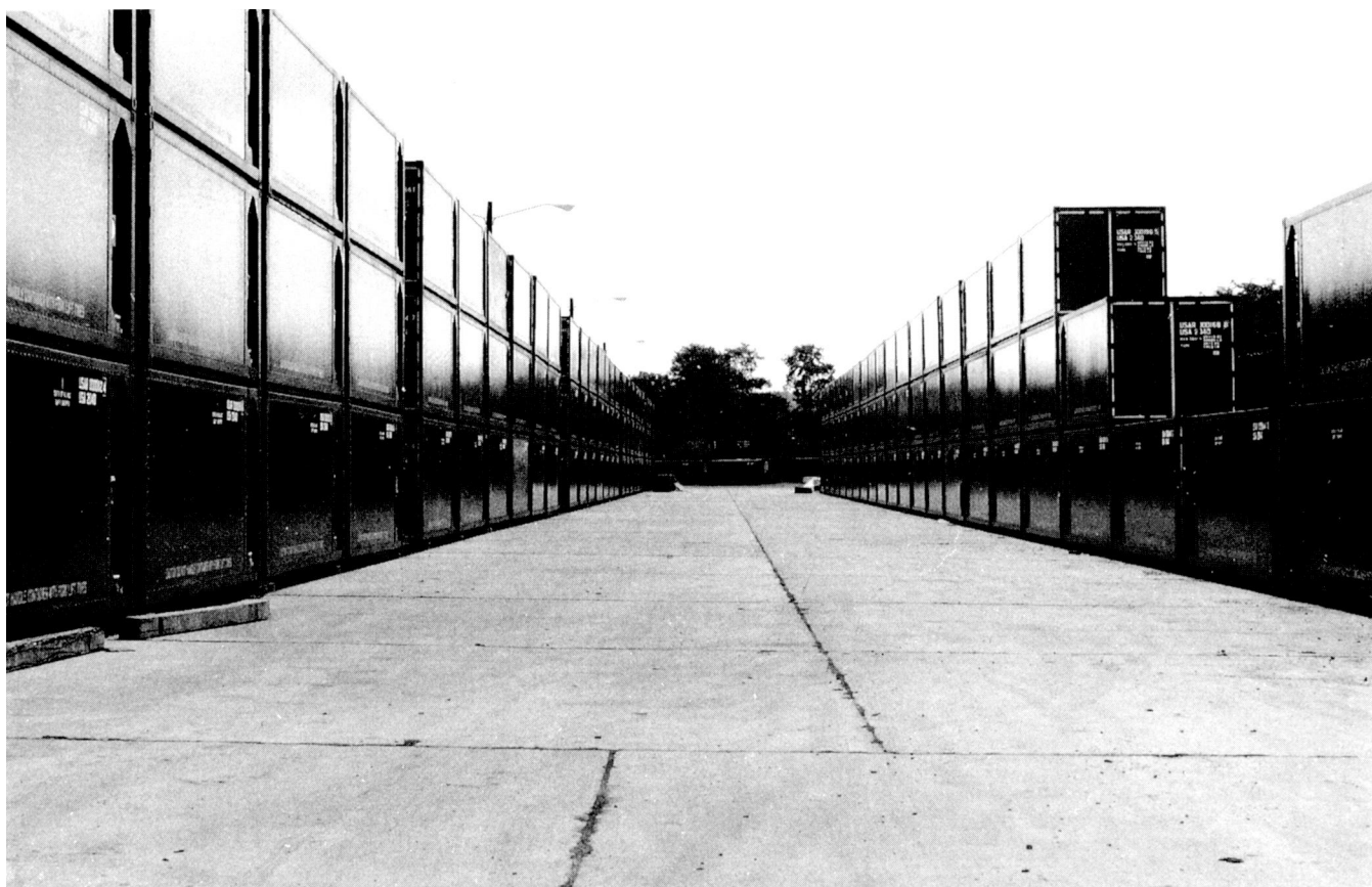
Figure 4-6. Containers stacked 3 high on concrete pavement.
