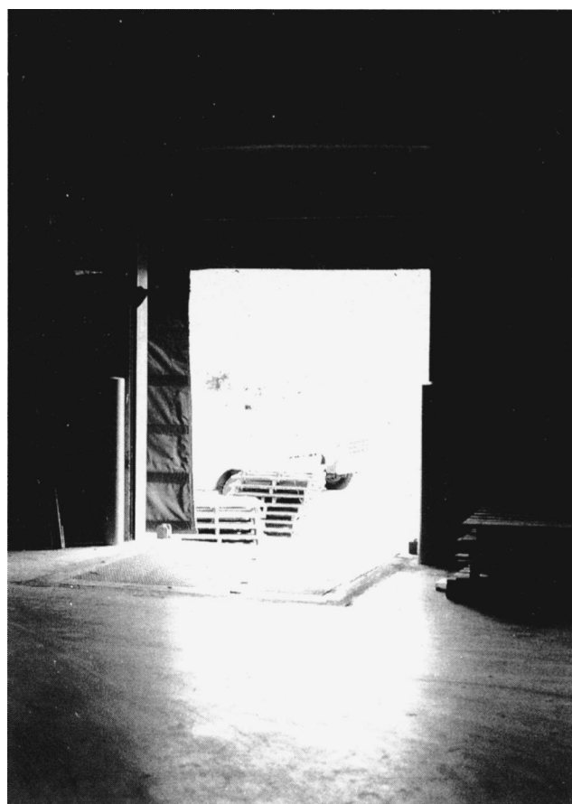
Figure 3-1. Hydraulic dock leveler.
