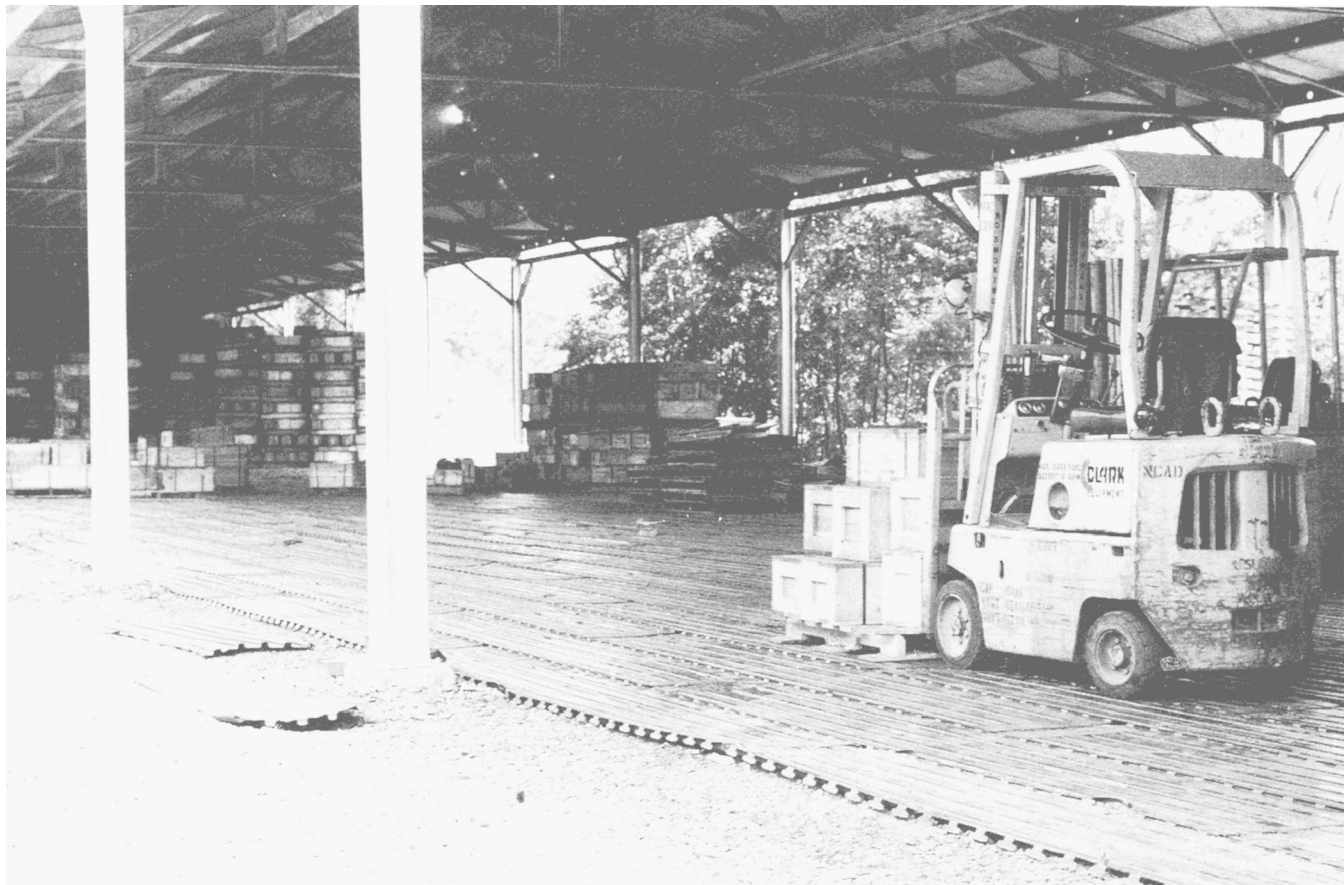
Figure 4-3. Flooring in shed area upgraded by use of steel military landing mats.
