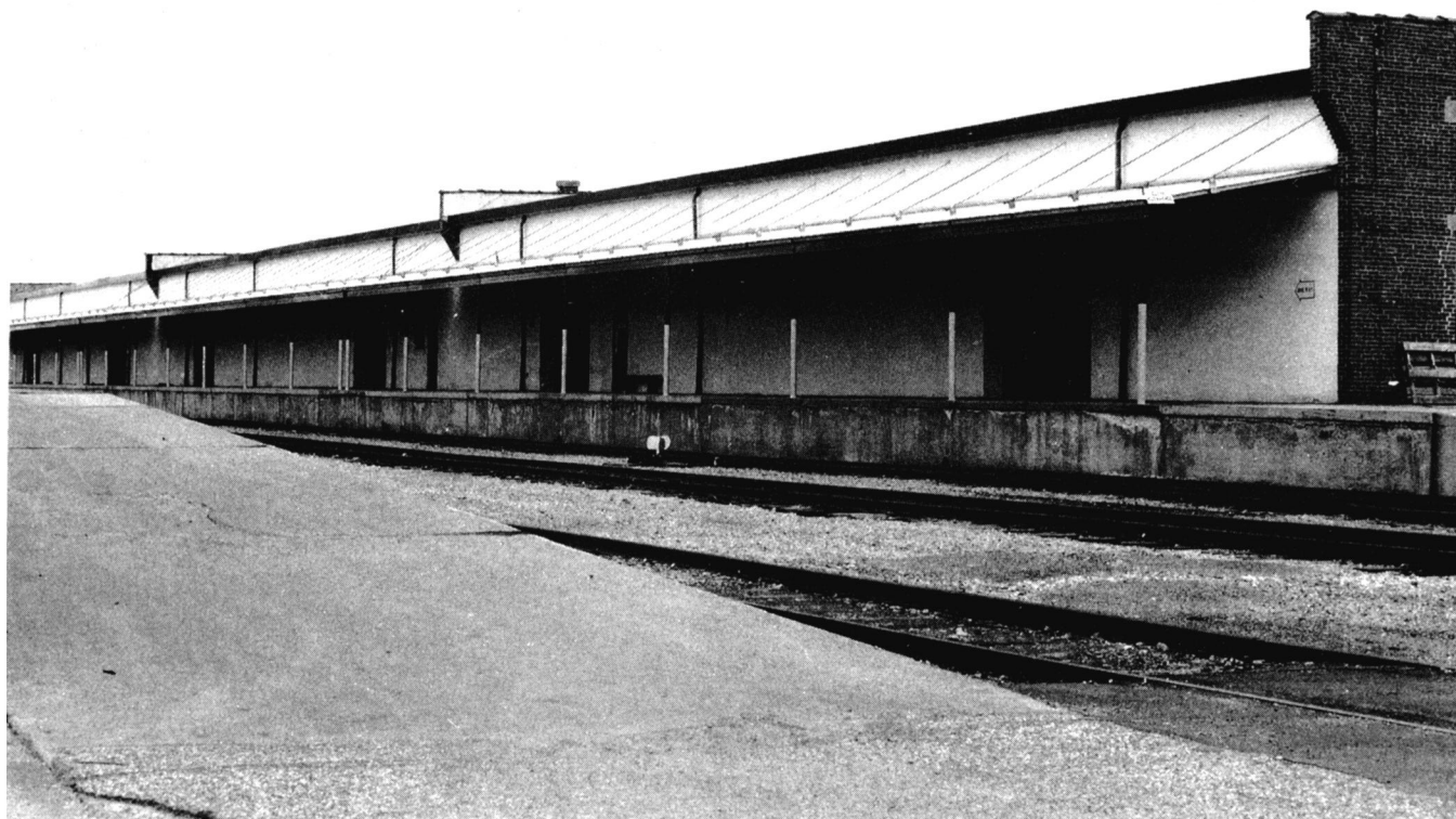
Figure 3-4. Covered exterior dock space.
