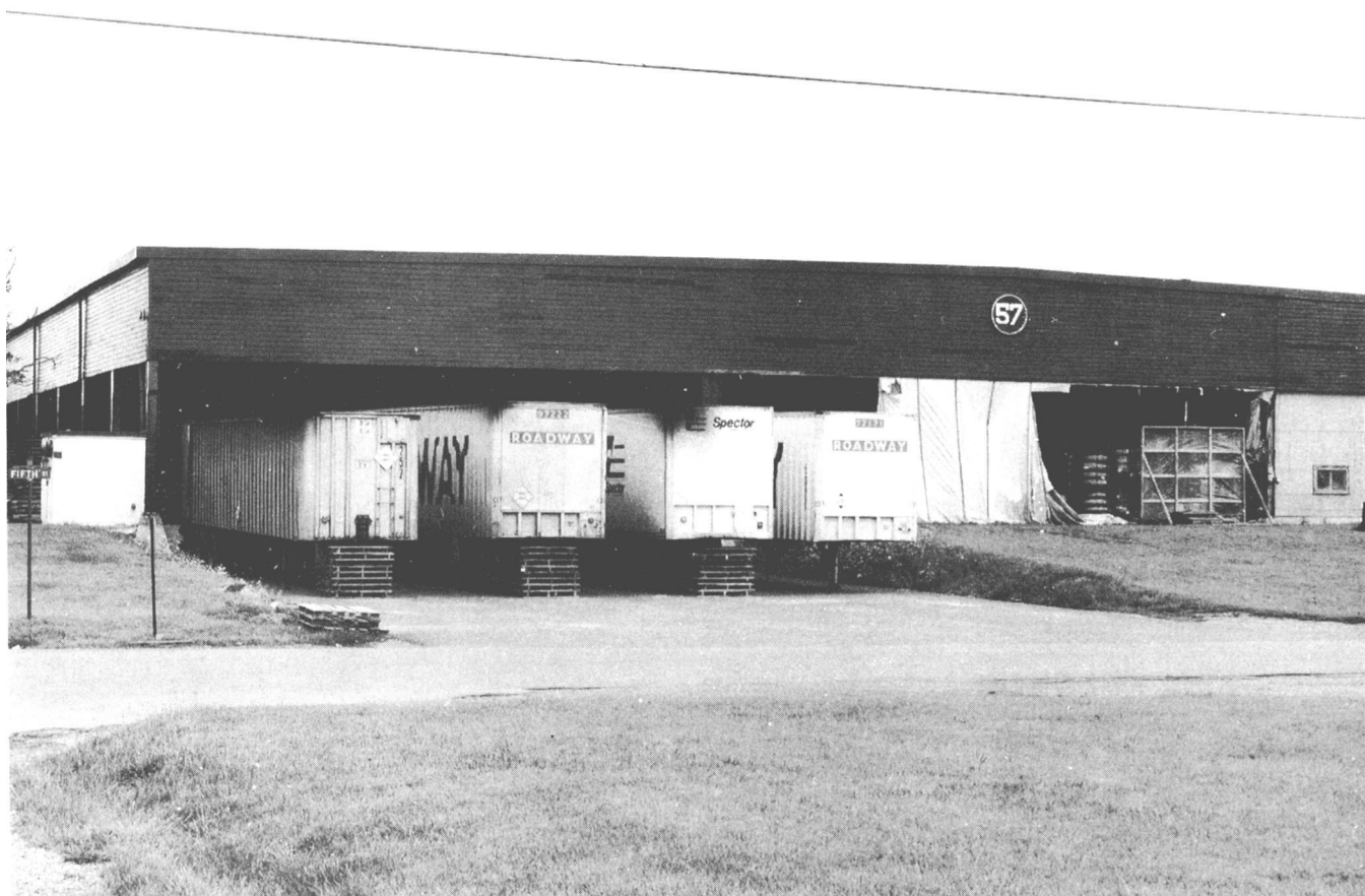
Figure 4-2. Storage shed with raised floor.
