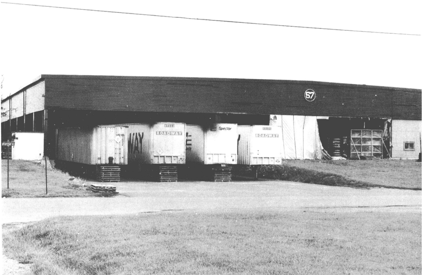
Figure 4-2. Storage shed with raised floor.
