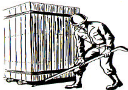
Figure 4-20. Use of wedge point bar and rollers
