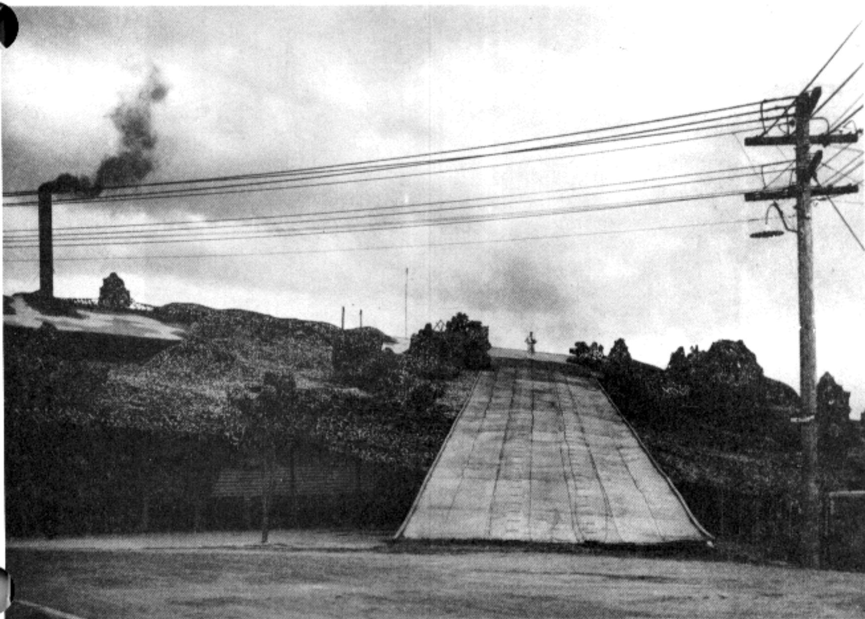
Figure 68. Ground view of a camouflaged mess hall of a munitions factory in Brisbane, Australia (1943). The false road continues on over the building and terminates logically at a route juncture. This is an excellent example of camouflaging a permanent installation.
