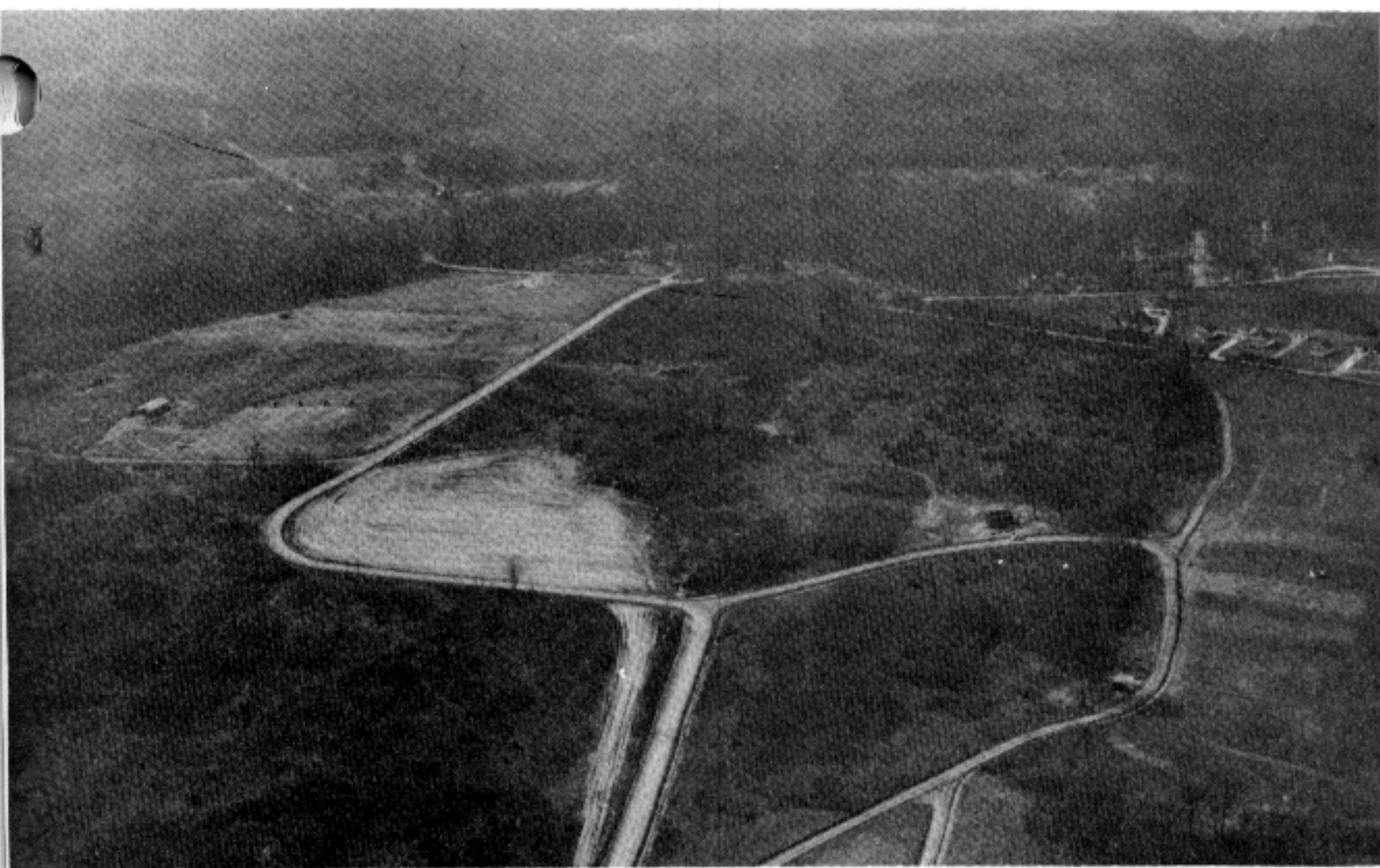
Figure 54. Careless and widespread earth scarring is caused by failure to establish a traffic plan, indiscriminate use of earthmoving equipment, and too much concern with leveling and clearing to facilitate construction. An enforced traffic plan, set up during the planning stage would eliminate much of the revealing scars in this picture.
