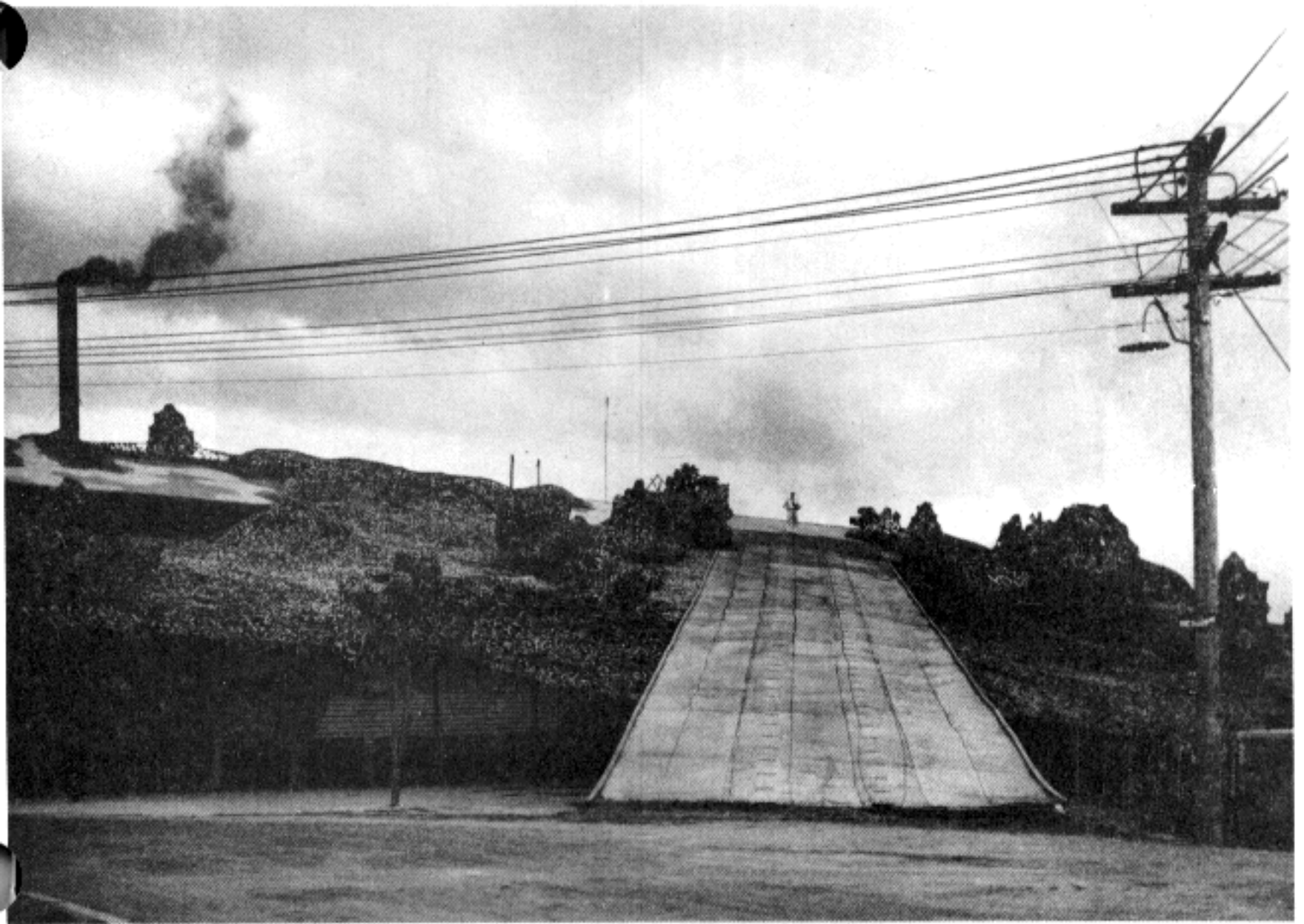
Figure 68. Ground view of a camouflaged mess hall of a munitions factory in Brisbane, Australia (1948). The false road continues on over the building and terminates logically at a route junction. This is an excellent example of camouflaging a permanent installation.
