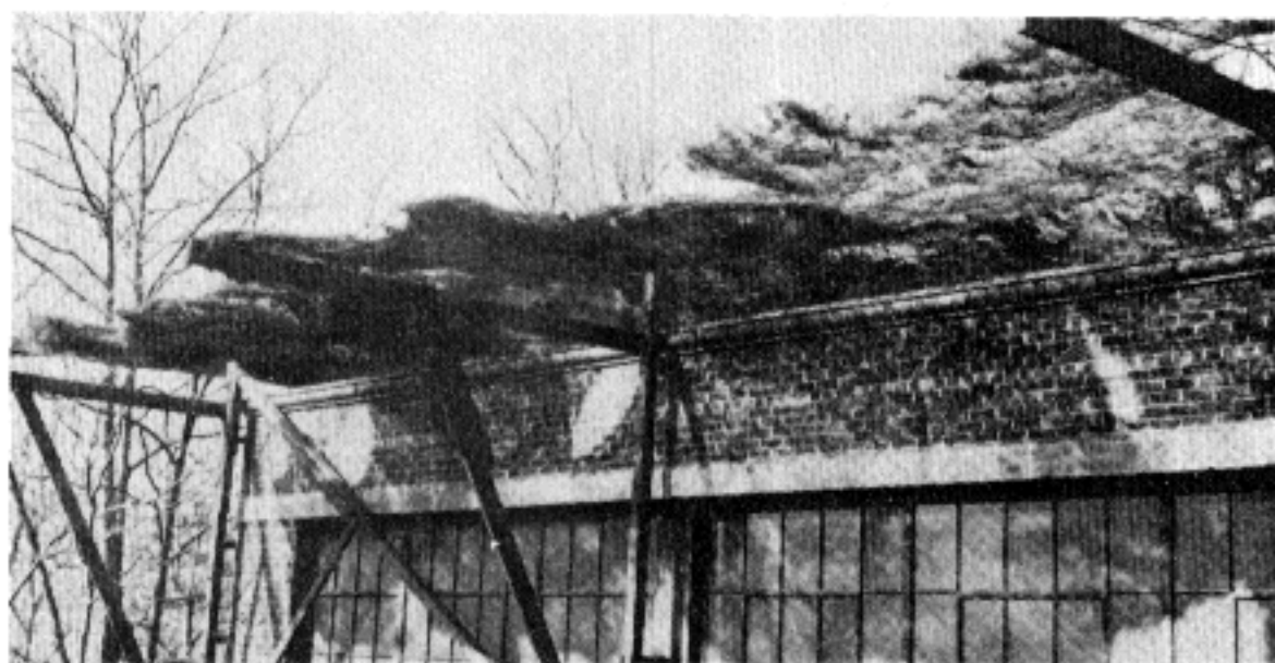
Figure 61. Netting garnished with steel wool distorts the shape of this building from aerial view.
