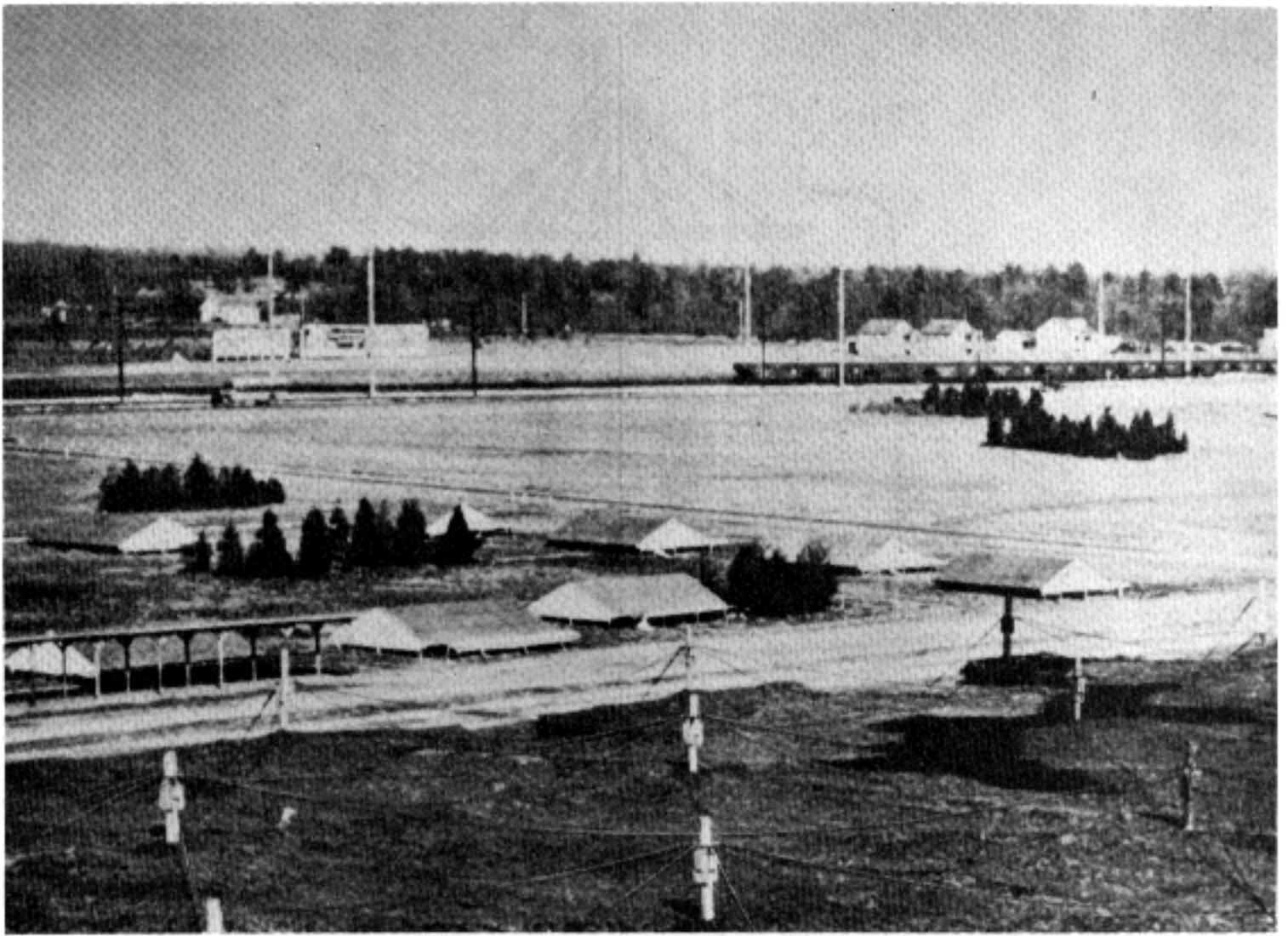
Figure 67. Disruptive pattern painting is used in conjunction with false structures. Houses similar to those in the background are simulated by three dimensional false roofs.
