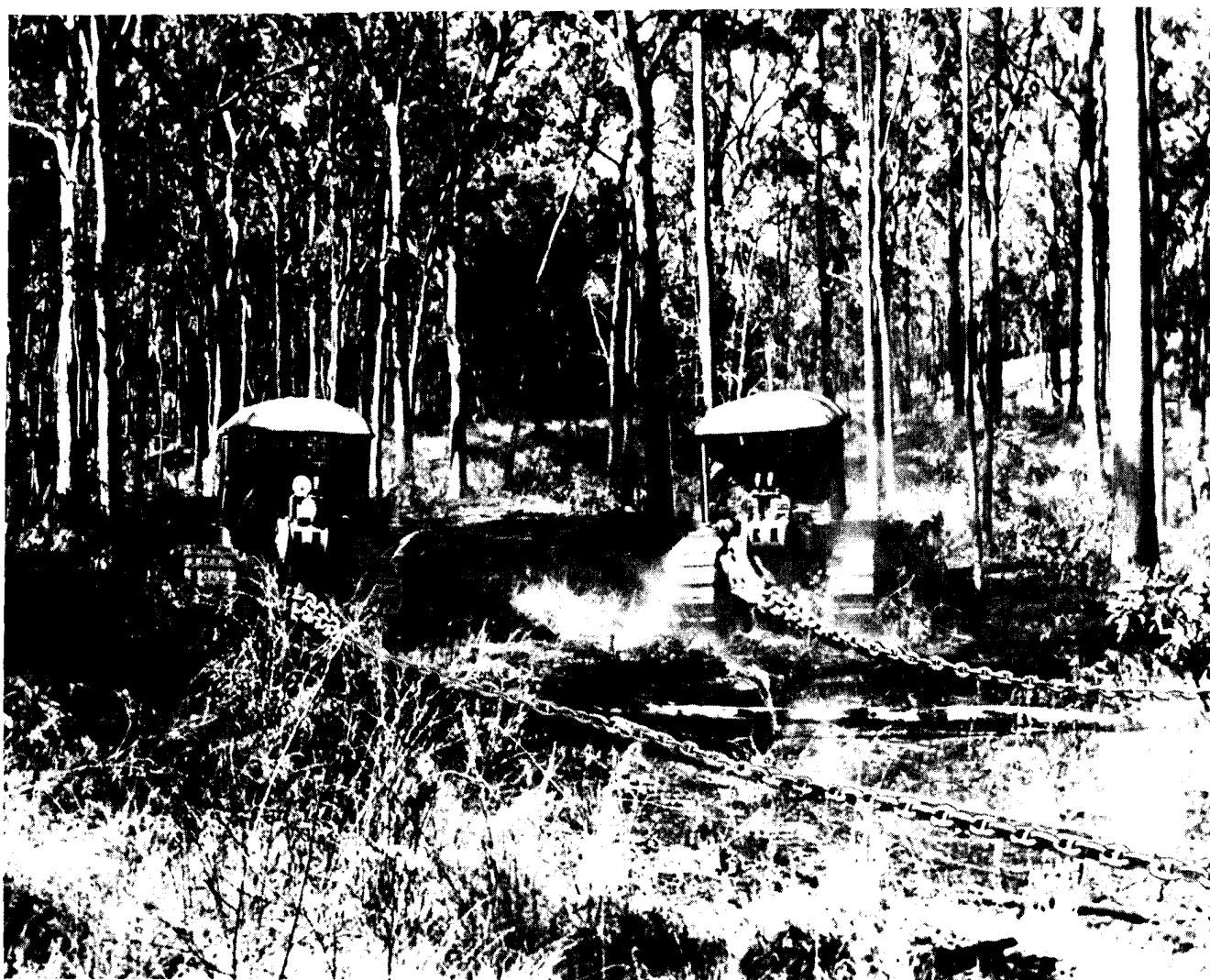
Figure 3-10. Two large crawler tractors towing anchor chain into clearing position.
