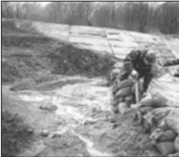
Figure 6-2. Digging a dike/berm.
