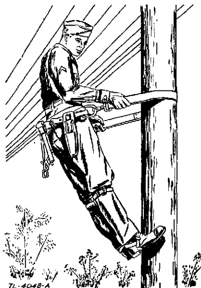
FIGURE 74.—Testing the safety belt.
