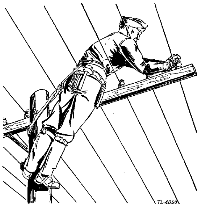
FIGURE 75.—Working on outer wire of cross arm.
