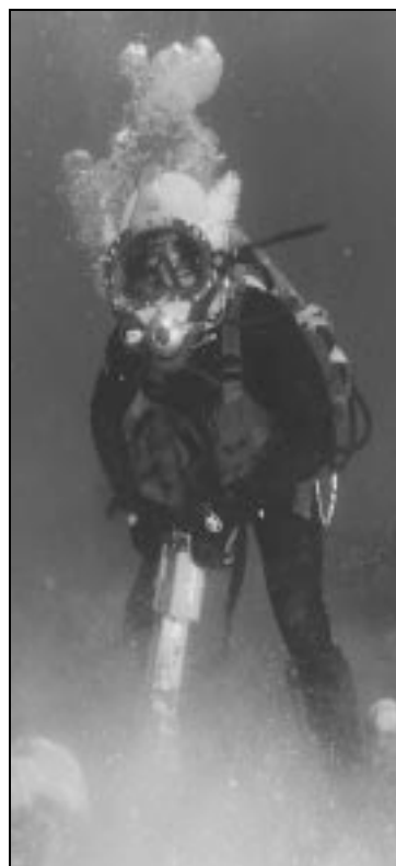
Figure 6-4. Underwater Construction Diving.
