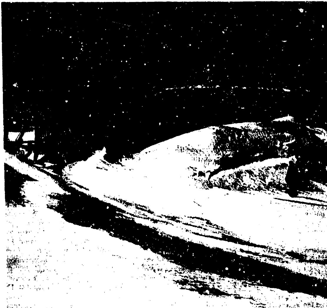
Figure 8-42. Snow Accumulation at a High Snow Fence (12-ft, wood slat drift fence erected permanently along a major highway in Northern Michigan. Note "blow-out" when a section of the fence was removed and not replaced to permit access to cultivated field.) (Photograph supplied by R. W. Gerds!)
