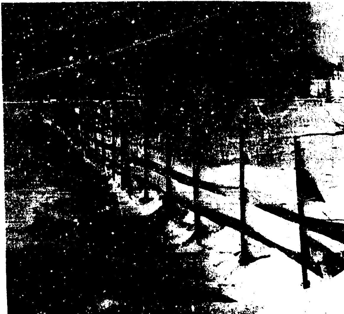
Figure 8-40. Paper Drift Fence (This is shown erected along a highway in Northern Michigan. Note that many more iron fence posts are used than normally required for the common wood slat fence.) (Photograph supplied by R. W. Gerdal)
