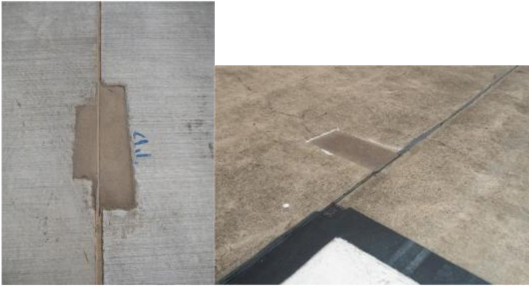
Examples of Semi Rigid Epoxy (SRE(S)) Repairs in Concrete Pavements
