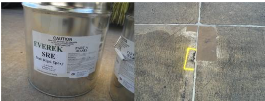
SRE(S) Repairs in Concrete Pavements
