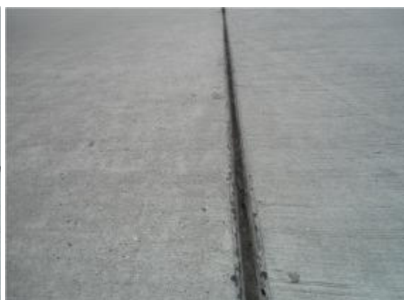
Chamfered Concrete Joint
