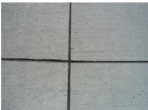
Example of "Good" Concrete Joint Sealing
