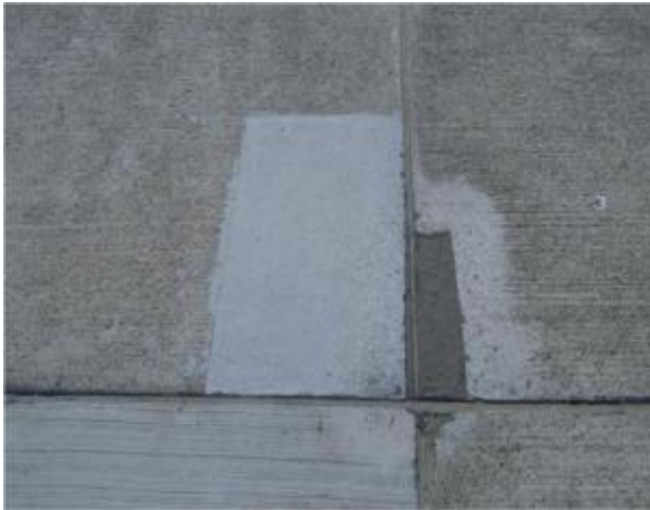
Example of “Good” Concrete Repair
